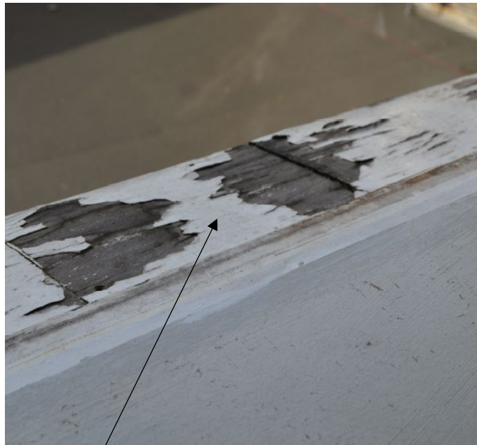
Detail of cill failure
