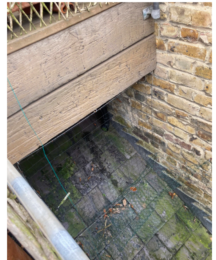
Roof decking structure sitting on top of existing roof - to be retained but reinforced to support new structure.
