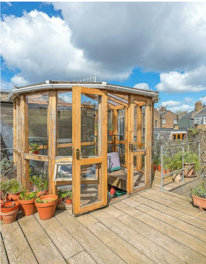
Single-glazed timber conservatory sitting on roof deck structure
