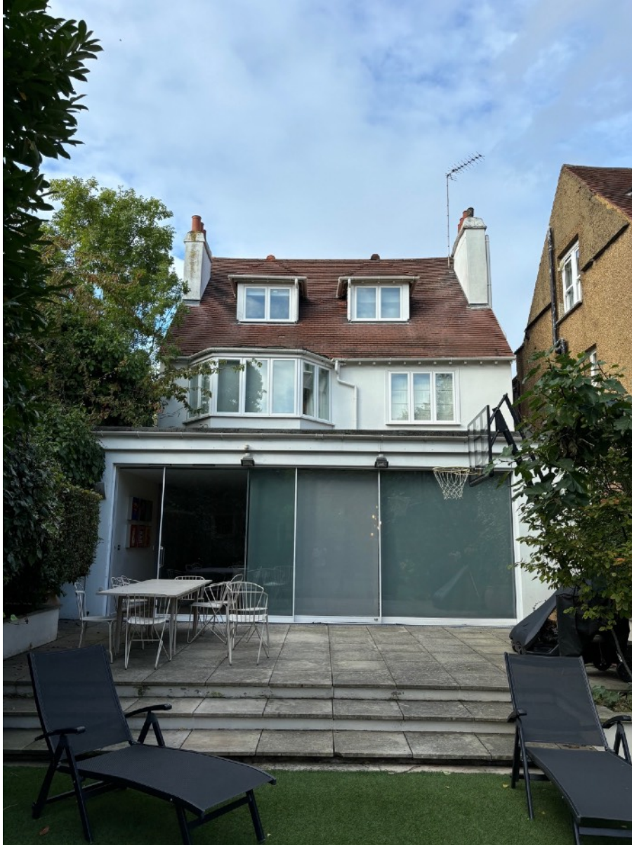
8.2. Fig 3. Existing Rear Elevation
