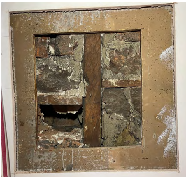
South wall of living room with panelling and stud wall exposed. Old wallpaper and void to no. 116 visible through hole.
