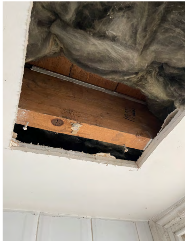
Bathroom flat roof joists, timber deck, loose insulation batts and plasterboard ceiling.
