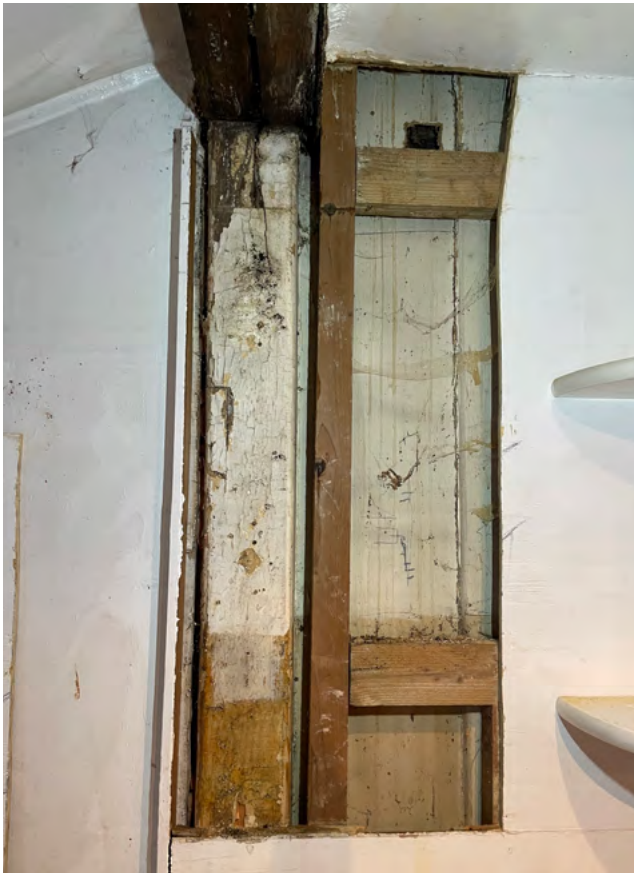
South wall, timber post and beam between main building and rear part of kitchen.
