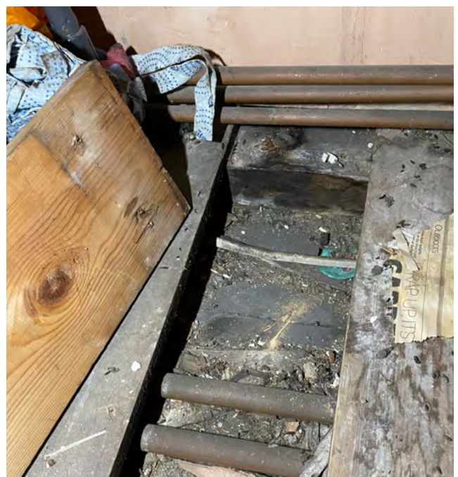
Kitchen floor within boiler cupboard, showing modern boards on bearers over service void with old boards below.
