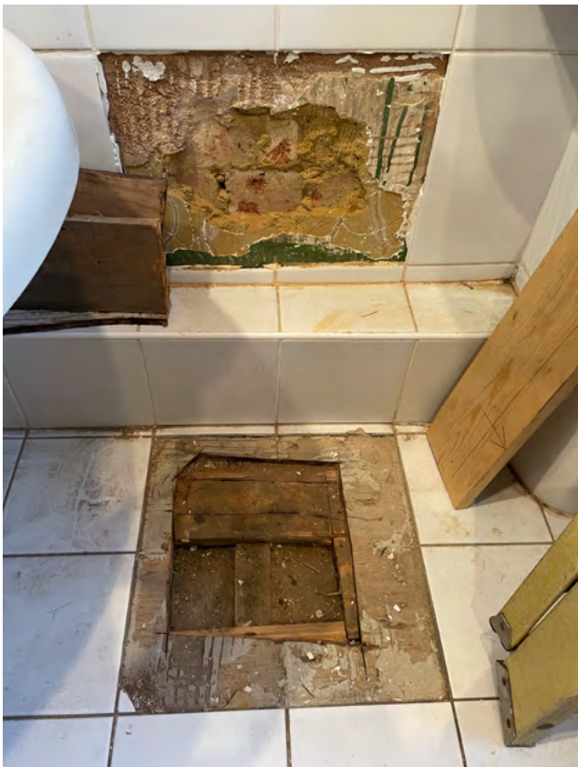
Bathroom wall construction (masonry rendered) and floor construction (firrings and boards over screed).
