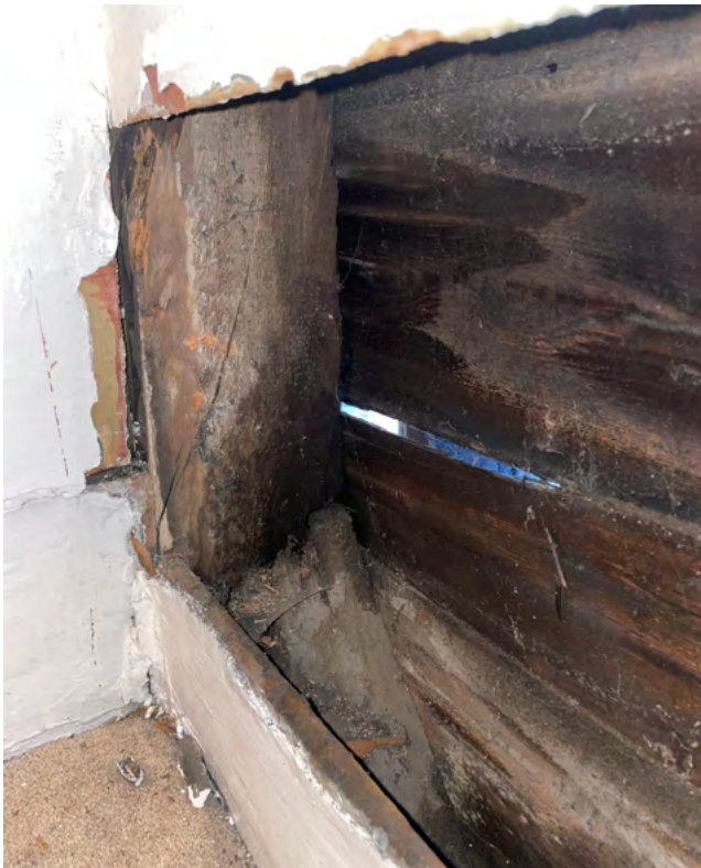
External wall to stair showing internal panelling, timber frame and external cladding.
