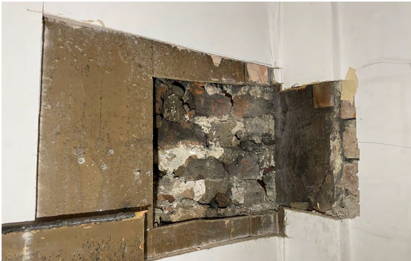
Junction of south wall (left) and west wall (right). Old panelling over stud wall with masonry infill. 120cm stud at corner.
