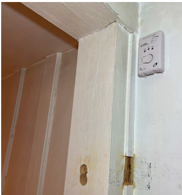
Cross-beam and post at north wall of kitchen. Timber post is a modern replacement.
