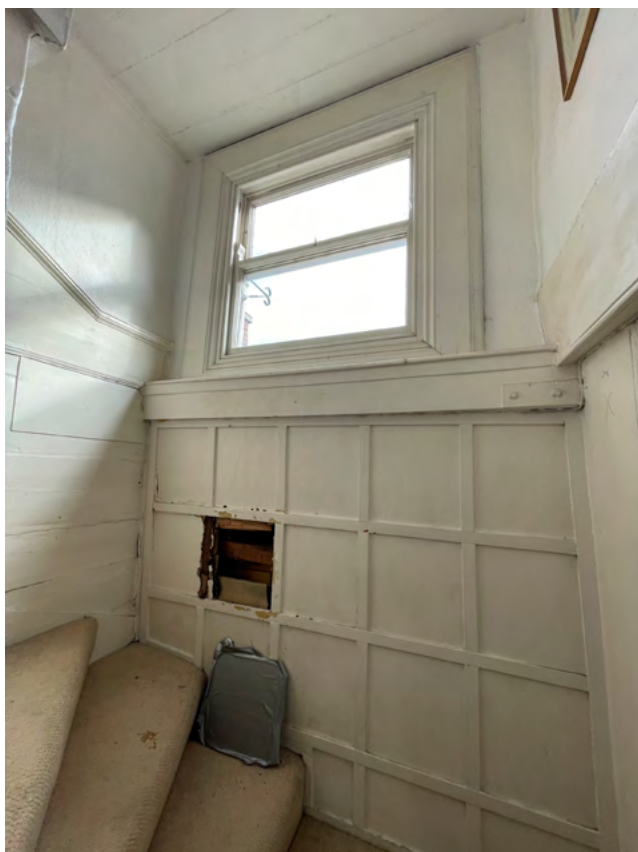
East wall with 20th Century panelling over old panelling.
