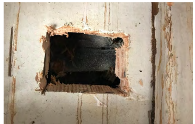
Plasterboard lining cut away to show old tongue and groove panelling behind. Hole in old panelling (below) reveals the party wall has a timber frame construction with timber panelling on either side. The frame is without brick infill.
