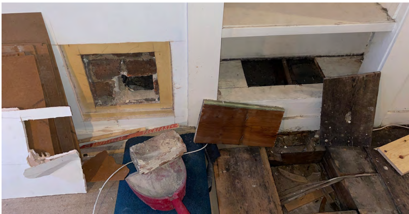
North wall of living room showing (left) timber stud wall with masonry infill and void behind, with cream coloured old timber panelling, and (right) floor joists extending below bookshelves to wall behind.
