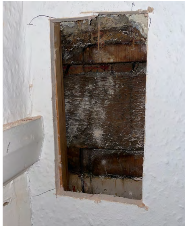
External wall to stair at southeast corner showing internal panelling, timber frame and external cladding.
