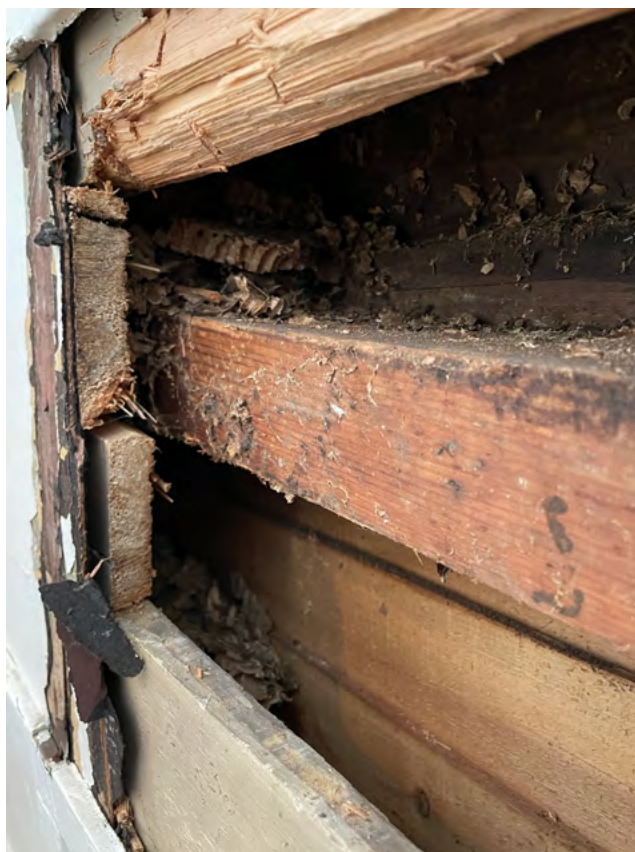
Two layers of panelling over frame; external weather boards.
