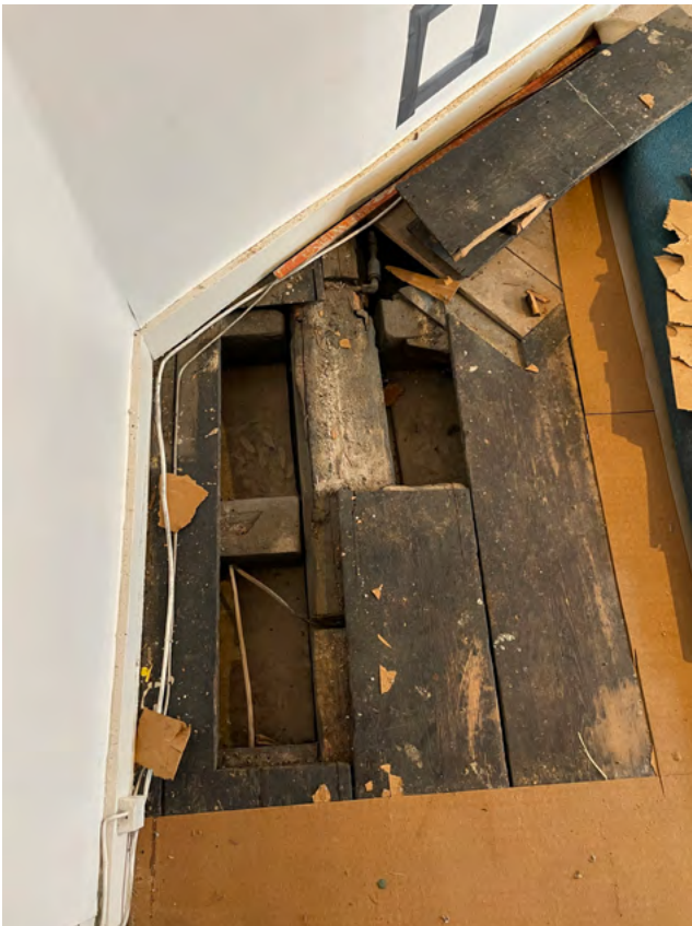
Close-up views of beam and joists showing condition and notching for services.
