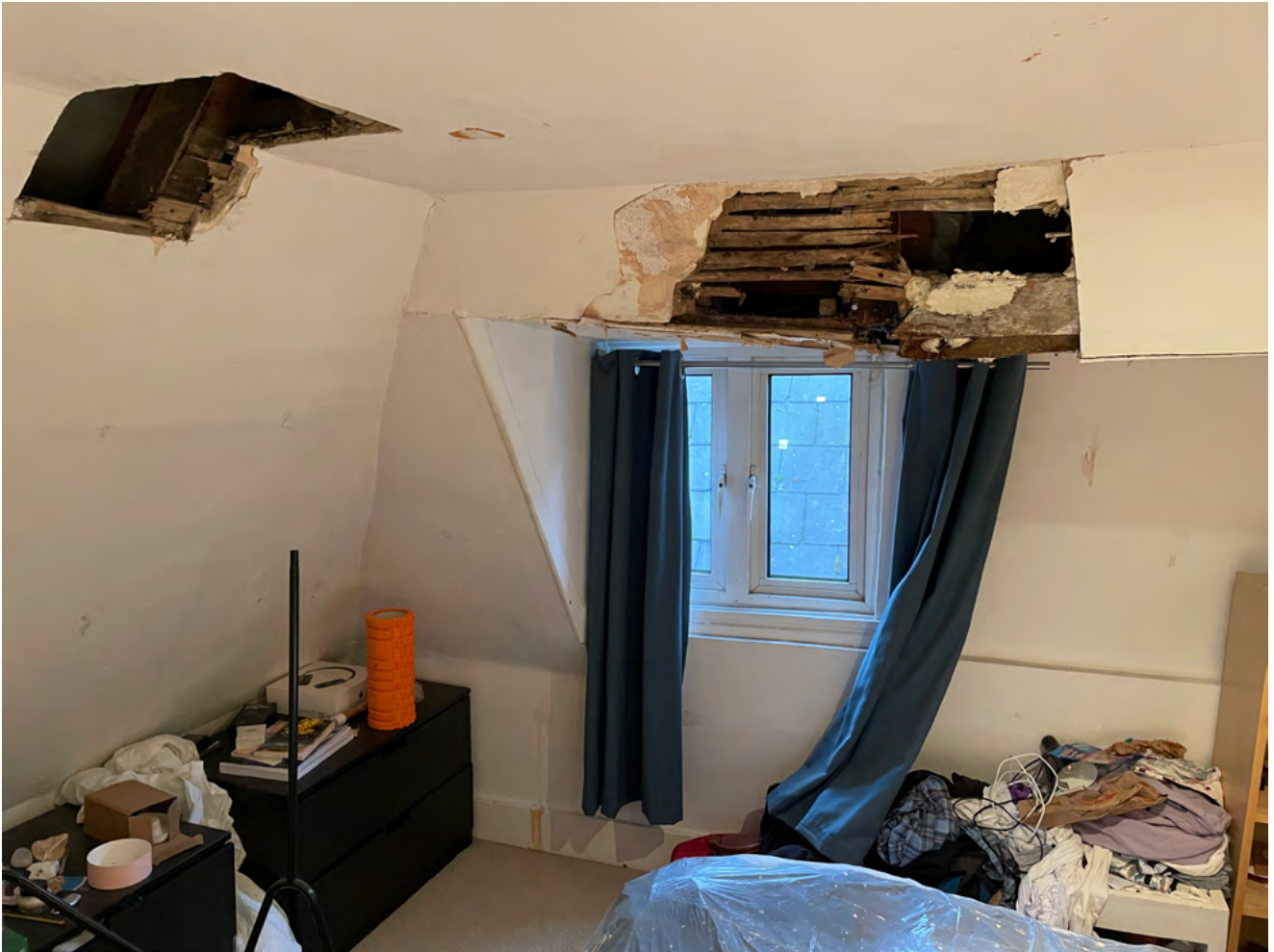
South and East walls opened, showing lath and plaster ceilings, and structural failure to south (side) dormer.
