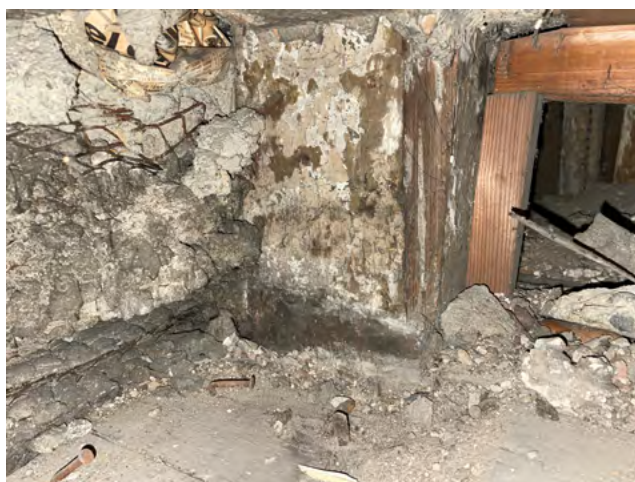
North wall floorboards and stud wall within wall void. Photograph on right shows concrete beam of no. 116 Heath Street.
