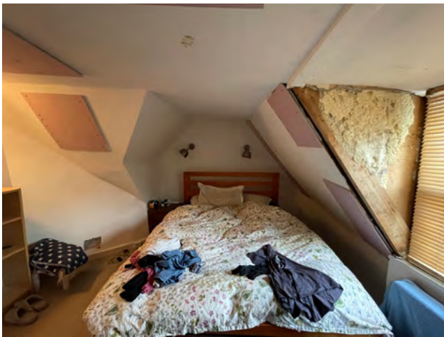
Facing south wall, showing exposed cheek of dormer.
