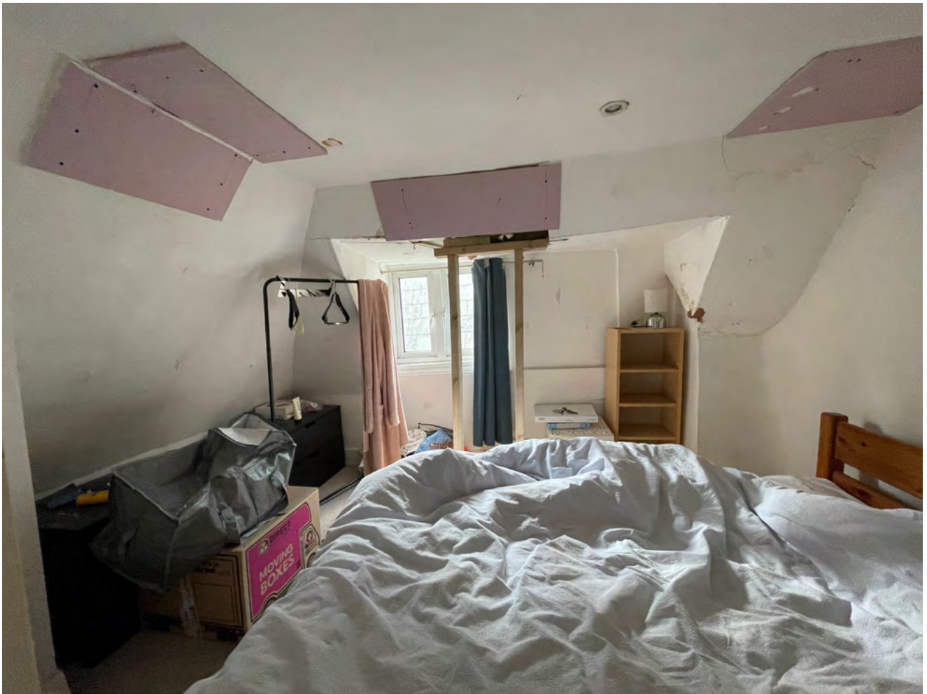
South wall showing interior of side dormer, propped due to structural failure.
