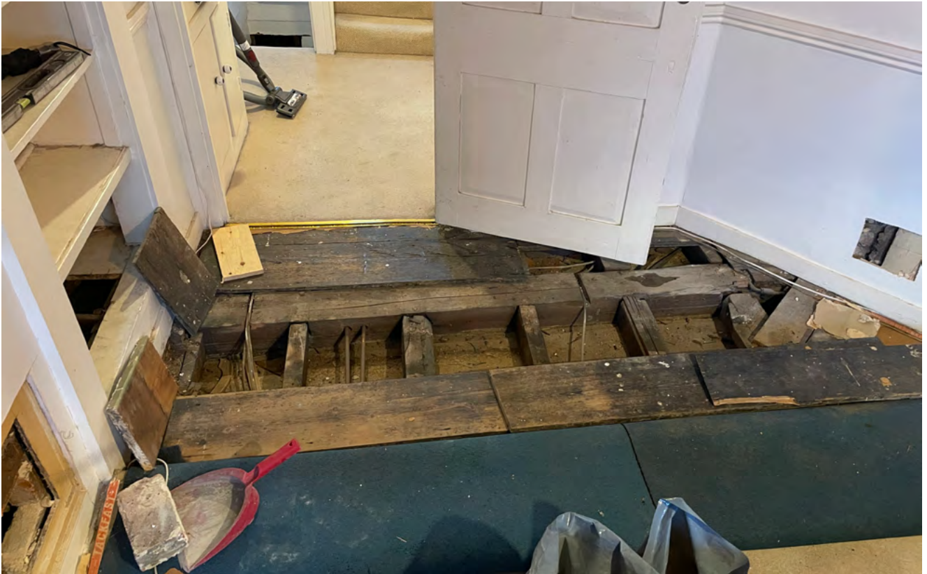
Living room floor construction: cross-beam between party wall and chimney stack, and joists between beam and front wall.
