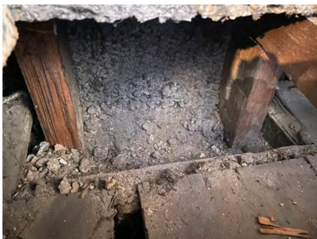
North wall floorboards and stud wall within wall void. Photograph on right shows concrete beam of no. 116 Heath Street.
