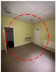
Wall will be demolished at 28 Woburn Square, London WC1H 0AA, UK to enlarge the space and used as class (Drawing no.12).
