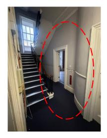
Wall will be demolished at 27 Woburn Square, London WC1H 0AA, UK to enlarge the space and used as class (Drawing no.12).
