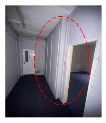
Wall will be demolished to enlarge the space and used as class (Drawing no.16).
