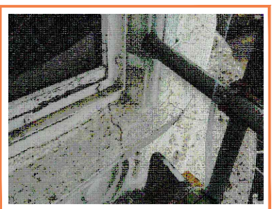
Photo 17 The rotten timber windows are to be sufficiently repaired or replaced to prevent further water ingress and degradation to the stone supporting cills and corbels. The cracks to the stonework around the windows are to be raked out and filled using a lime based stone repair mortar.
