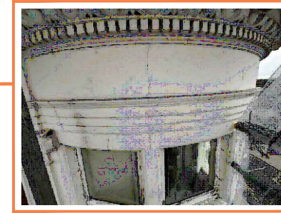
Photo 15 The cracks to the upper stone corbel are to be raked out and filled using a lime based stone repair mortar.
