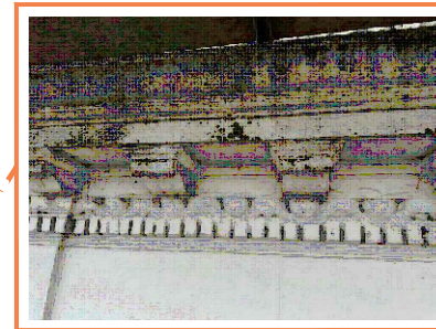
Photo 14 The cracks to the upper stone corbel are to be raked out and filled using a lime based stone repair mortar.
