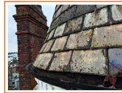
Photo 5 Any damaged or cracked tiles are to be carefully removed and replaced on a like for like basis.
