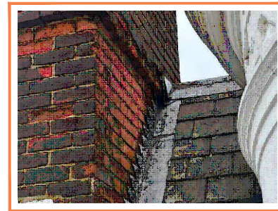
Photo 12 Existing lead flashing is to be secured back to the existing brickwork using an appropriate lead sealant.
