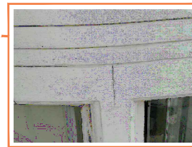
Photo 19 The rotten timber windows are to be sufficiently repaired or replaced to prevent further water ingress and degradation to the stone supporting cills and corbels. The cracks to the stonework around the windows are to be raked out and filled using a lime based stone repair mortar.
