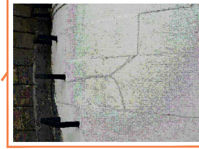
Photo 13 The cracks to the upper stone walls are to be raked out and filled using a lime based stone repair mortar.
