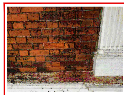
Photo 23 Blown/damaged bricks are to be sufficiently repaired using a brick masonry repair filler.
