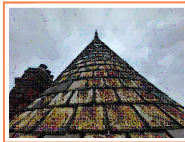
Photo 4 Any damaged or cracked tiles are to be carefully removed and replaced on a like for like basis.
