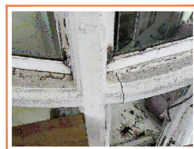
Photo 20 The rotten timber windows are to be sufficiently repaired or replaced to prevent further water ingress and degradation to the stone supporting cills and corbels. The cracks to the stonework around the windows are to be raked out and filled using a lime based stone repair mortar.
