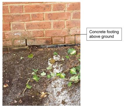
Photo 3: Wall Foundations at or Above Ground Level
