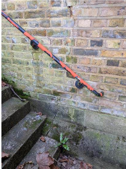
Crack in external wall
