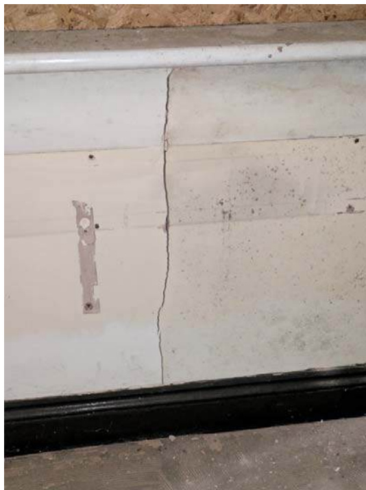
Crack under window in rear rooms
