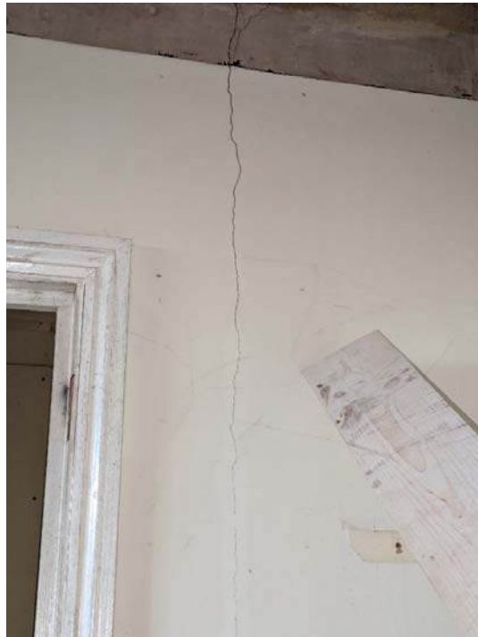
Crack in wall in rear room at first floor
