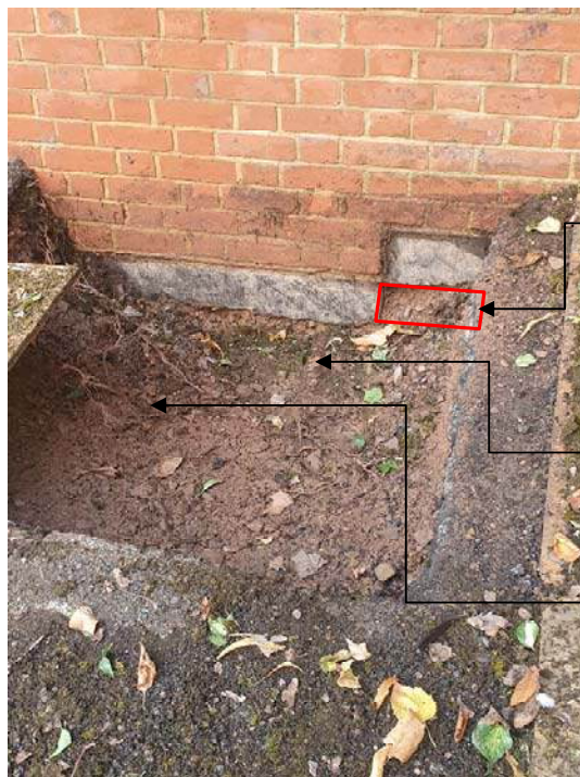
Photo 2: Trial Pit - Wall Foundations
