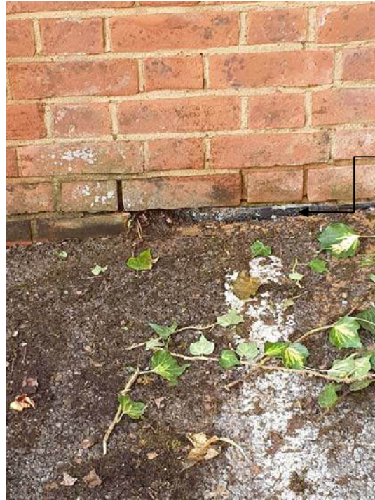
Photo 3: Wall Foundations at or Above Ground Level
