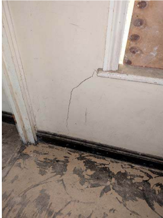
Crack adjacent to window in top landing
