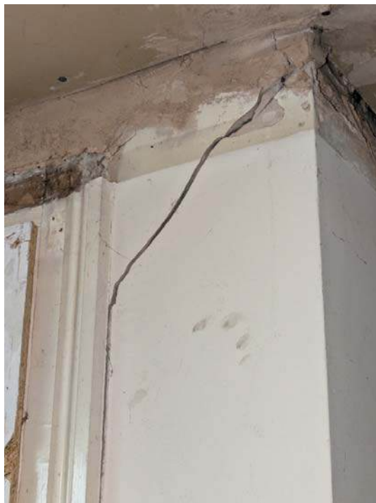
Crack in wall adjacent to bay window
