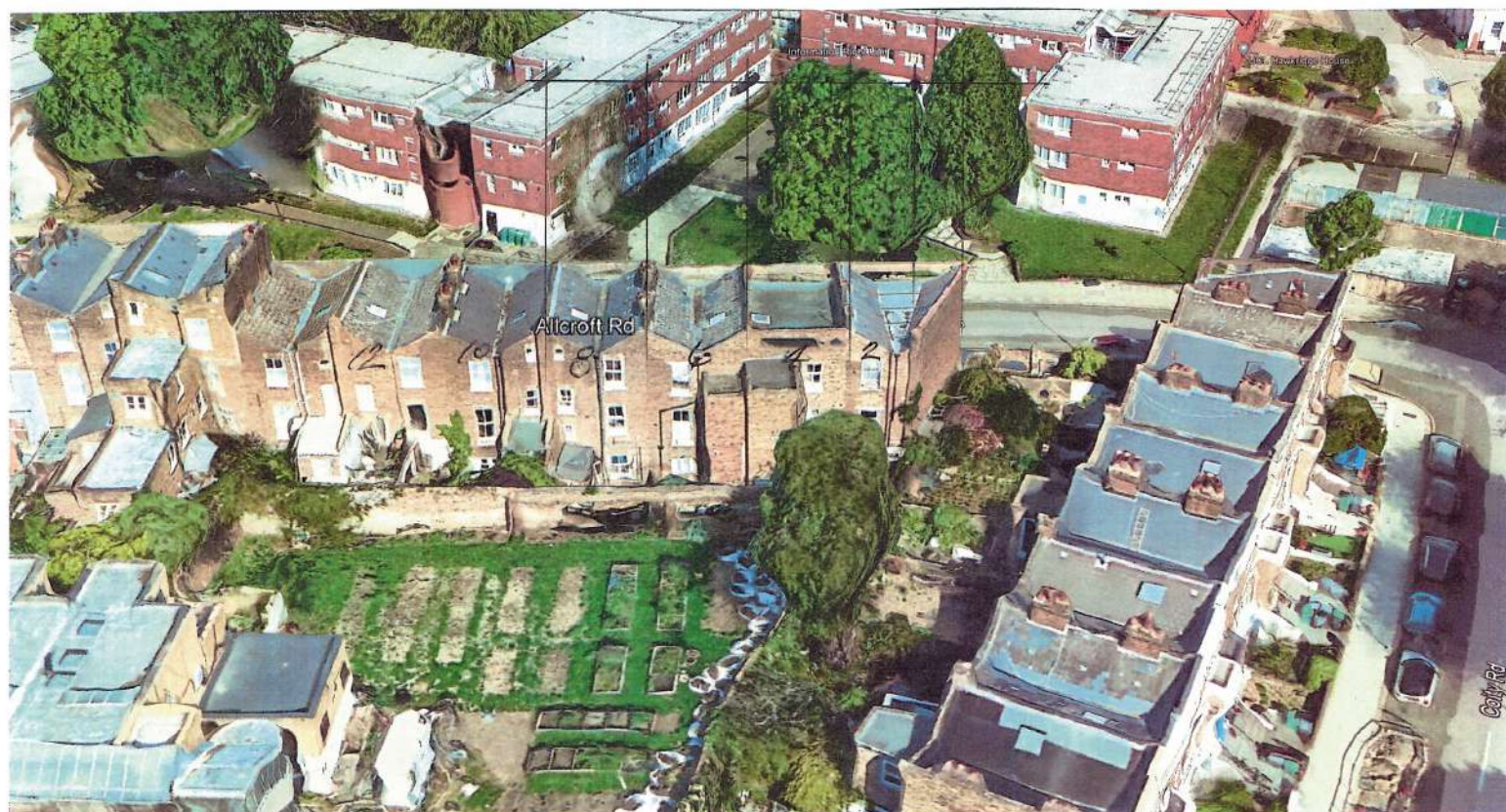
'AERIAL VIEW OF REAR OF ALLCROFT ROAD PROPERTIES'
