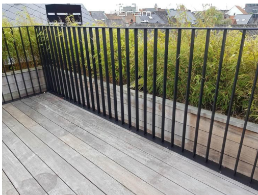
Figure 1 – Illustration only - Black metal railings fixed to masonry on terrace parapet
