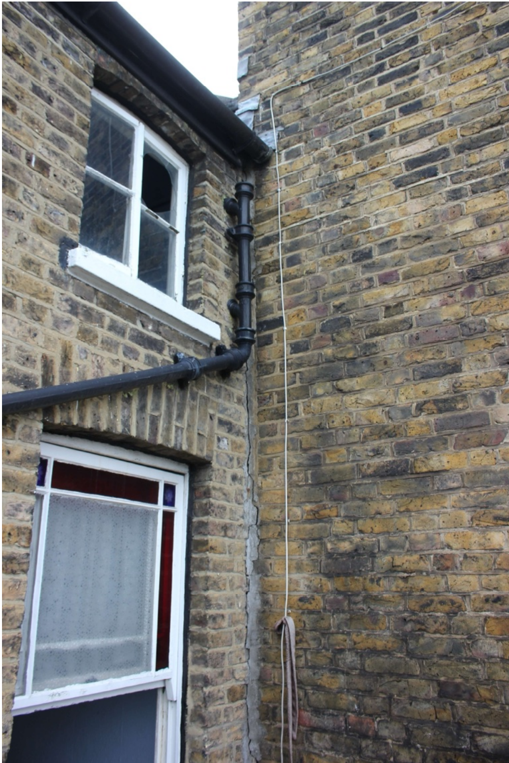
Photo 7 – Previously filled and open joints between the rear main wall and tall chimney
