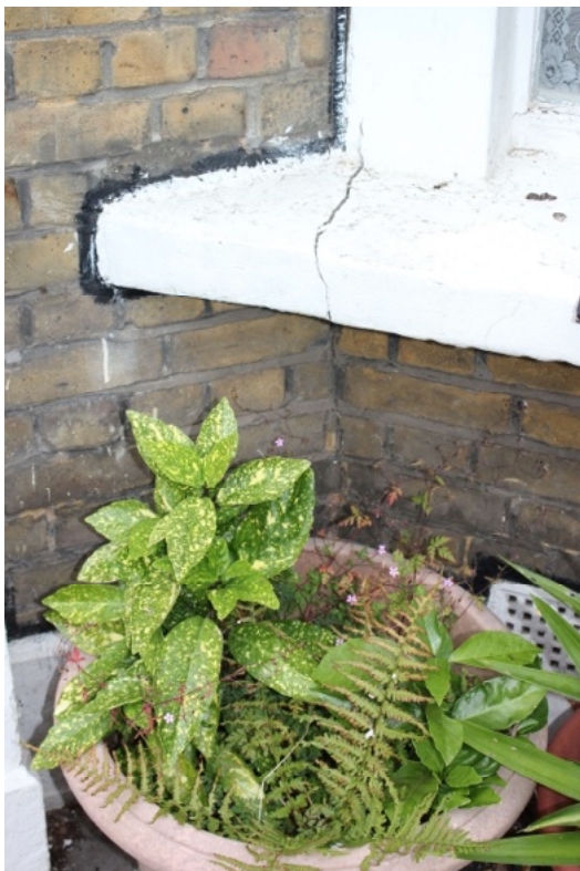
Photo 11 – Cracked bay sill
