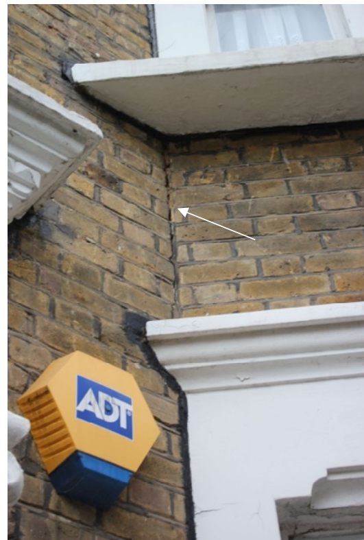
Photo 12 – Crack at bay wall junction
