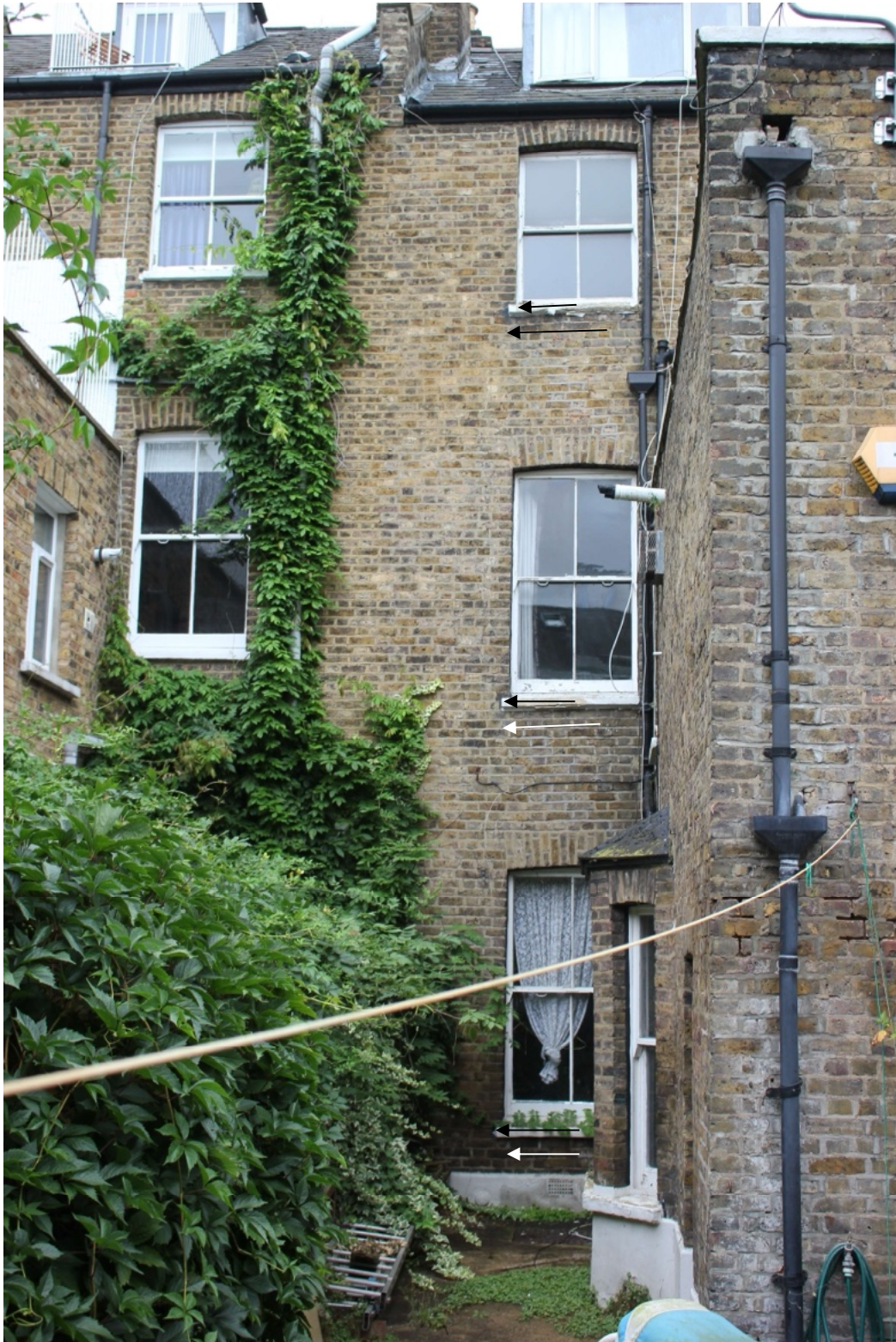
Photo 10 – Settlement of the rear main wall
