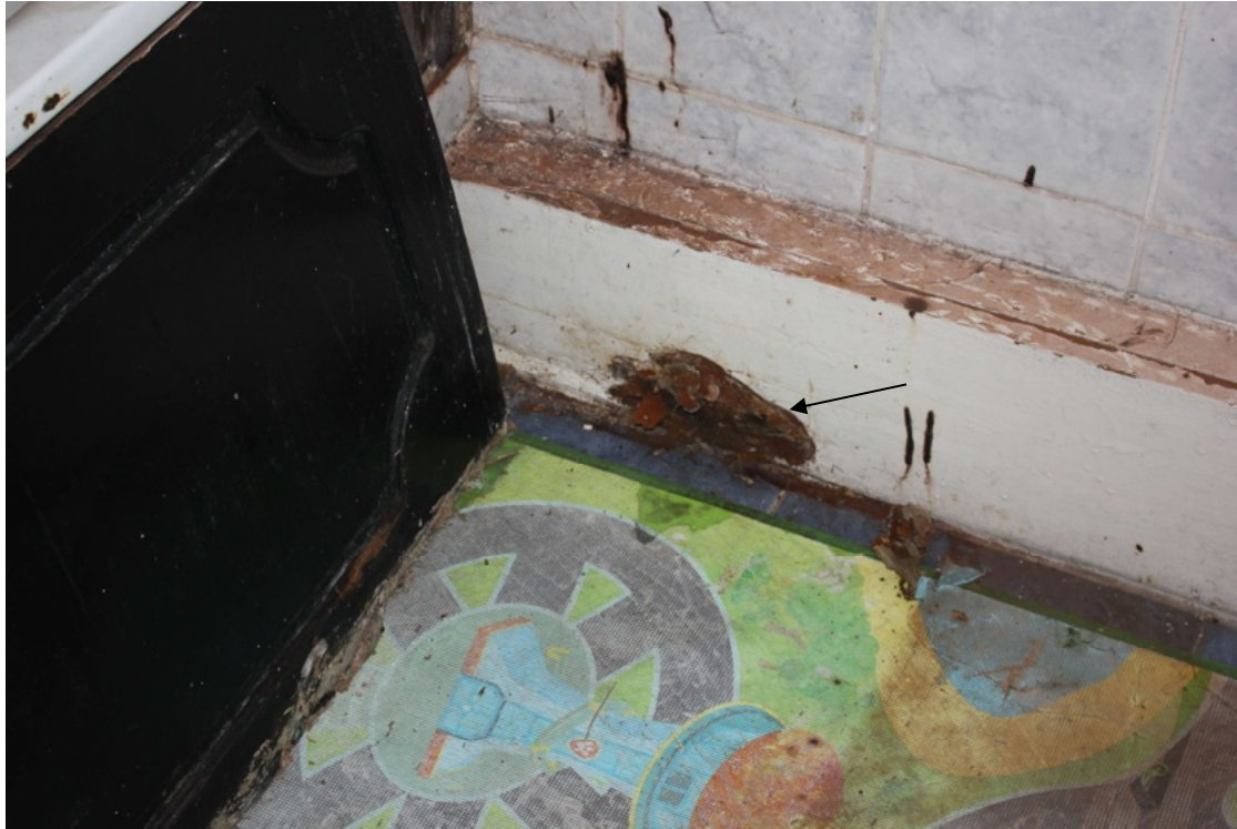
Photo 14 – Dry rot in the skirting board to the first-floor bathroom.
