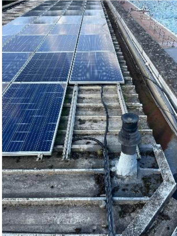
Existing Photovoltaics over the female changing rooms showing PV on spreader channels, cables hidden against parapet and PV avoiding existing roof penetrations
