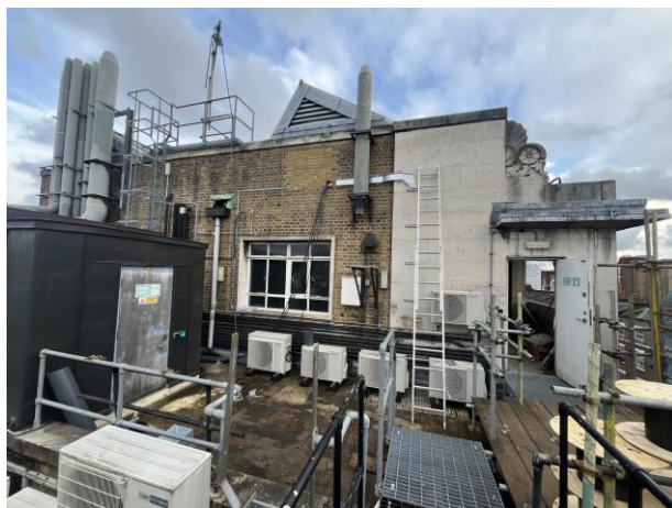
Image 2 replacement condenser units.
