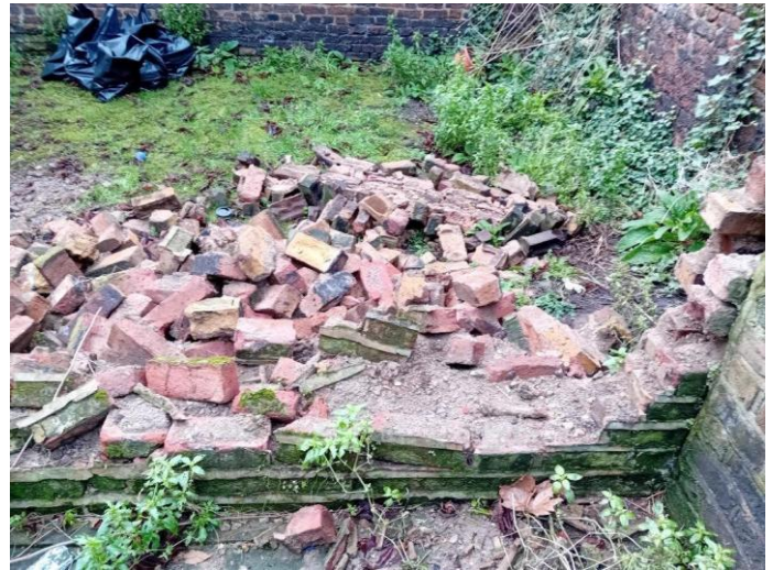
End of West Boundary wall (Collapsed)
