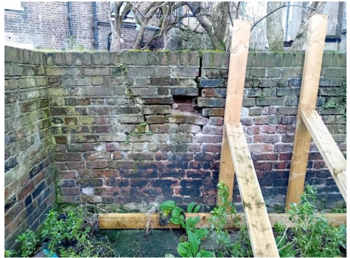
End of East Boundary Wall in poor condition with propping.
