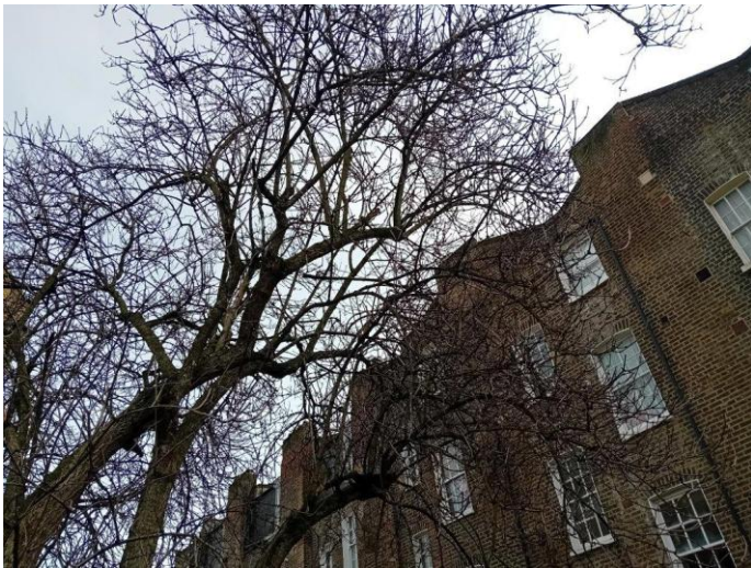
Neighbouring tree likely to be causing ground movement
