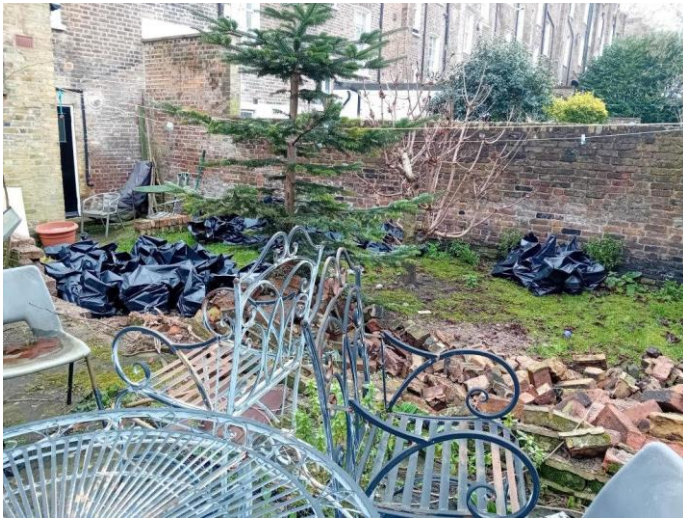
West Boundary Wall (missing, collapsed on to the floor)
