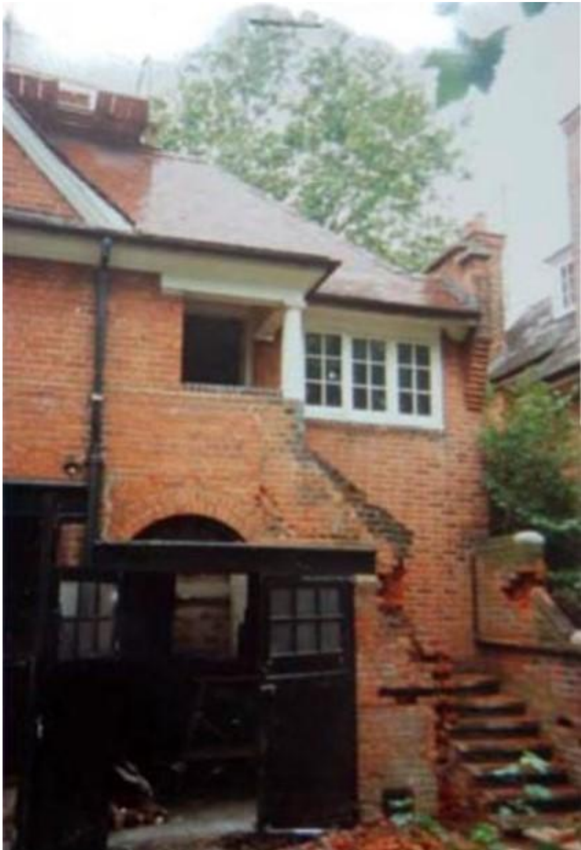
Fig 14: The photo shows the building under conversion in the 1980's with a pair of smaller garage doors in the side opening and the brickwork to the first floor staircase badly damaged and now subsequently rebuilt.
