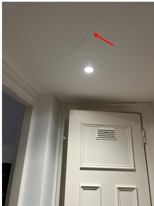
Photograph 12 – Cracking to ceiling
