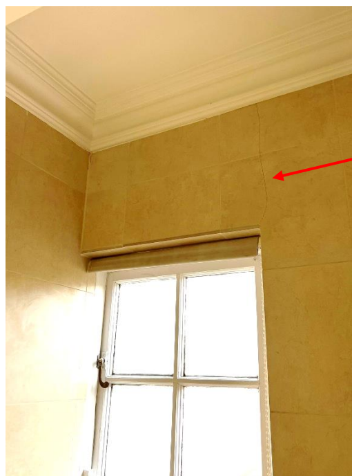
Photograph 10 – Crack to tiling in bathroom
