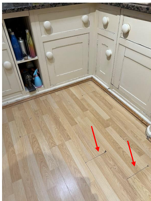
Photograph 9 – Opening up of flooring in kitchen
