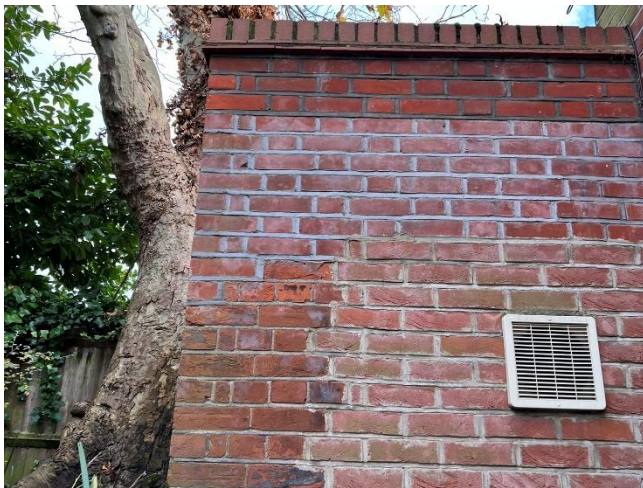
Photograph 3 – Trunk less than 300mm from rear wall of building
