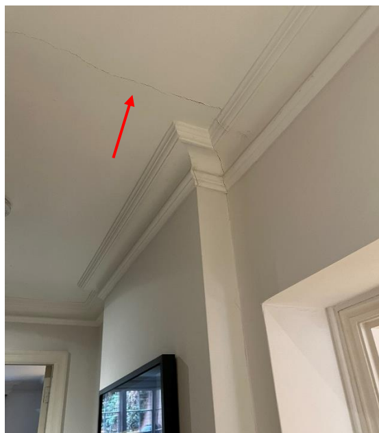
Photograph 14 – Cracking to ceiling
