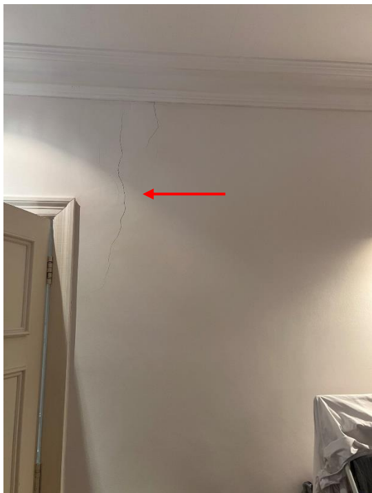
Photograph 11 – Cracking to wall
