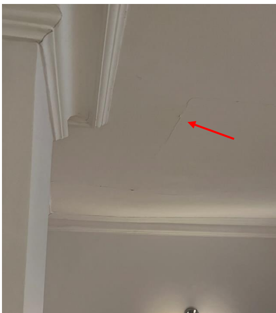
Photograph 13 – Cracking to ceiling
