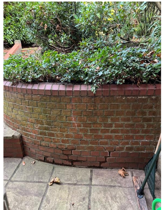
Photograph 6 – Cracking to retaining wall
