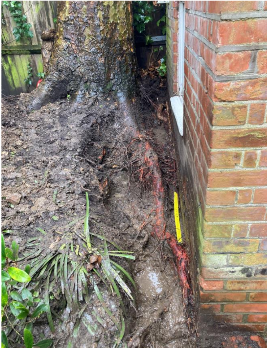
Photograph 2: showing the significant proximity between structural root of tree no. 1 and the rear extension wall of the listed building.
