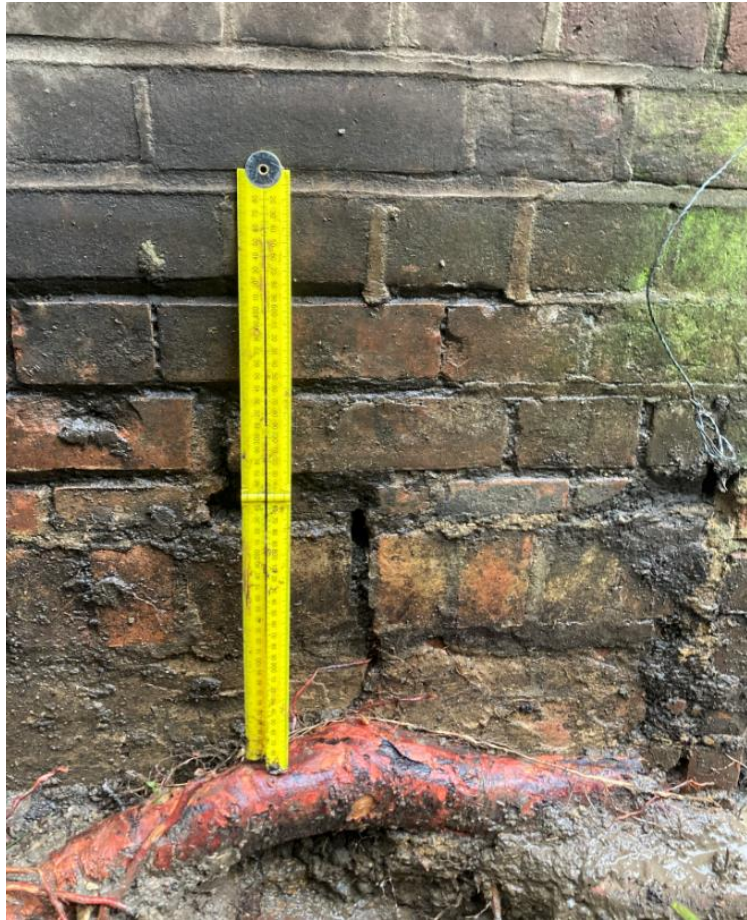
Photograph 4: showing the point at which the structural root grows directly against the rear extension wall; note the crack within the brickwork directly above.
