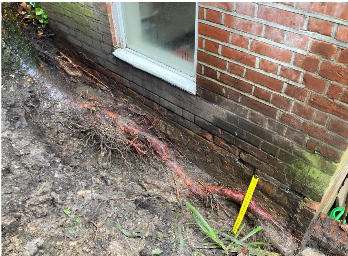
Photograph 3: showing the significant proximity between structural root of tree no. 1 and the rear extension wall of the listed building.
