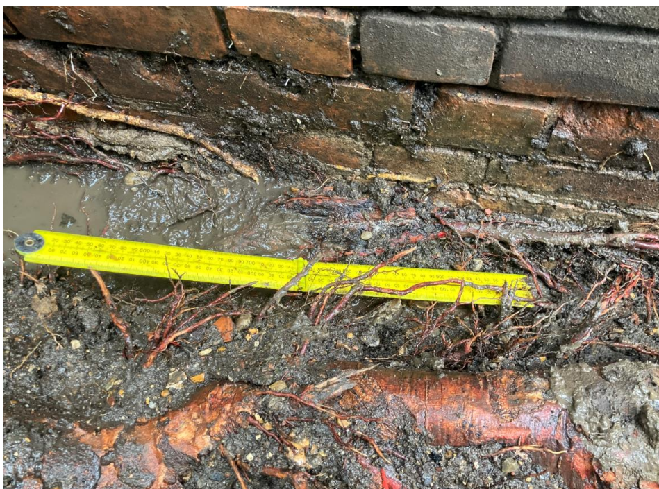
Photograph 5: showing the upper surface of an additional structural root that we were unable to fully excavate due to the density of roots, growing directly against the rear extension wall.
