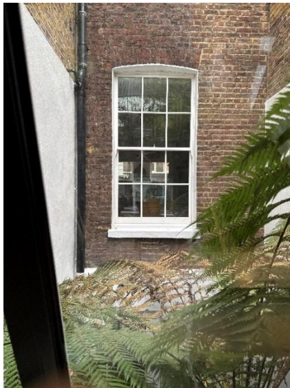
Image showing timber sash windows at rear of historic original part of building at ground floor looking into the courtyard
