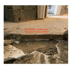
A professional assessment confirmed that failure to address the damp issue would lead to further deterioration of the internal living conditions.
