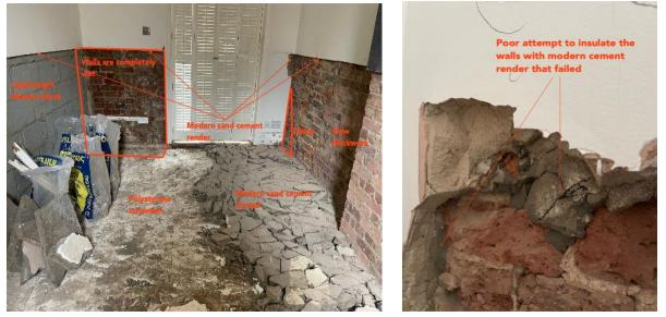
Moisture was rising through the screed, due to the lack of a functioning damp-proof membrane (DPM).
