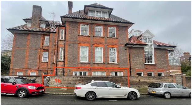
Flat 1B has its own separate ground-floor entrance from Hampstead Hill Gardens, while the main entrance for the rest of the flats is on Rosslyn Hill. The flat is situated approximately 600mm below external ground level, which has significantly contributed to the damp issues.
