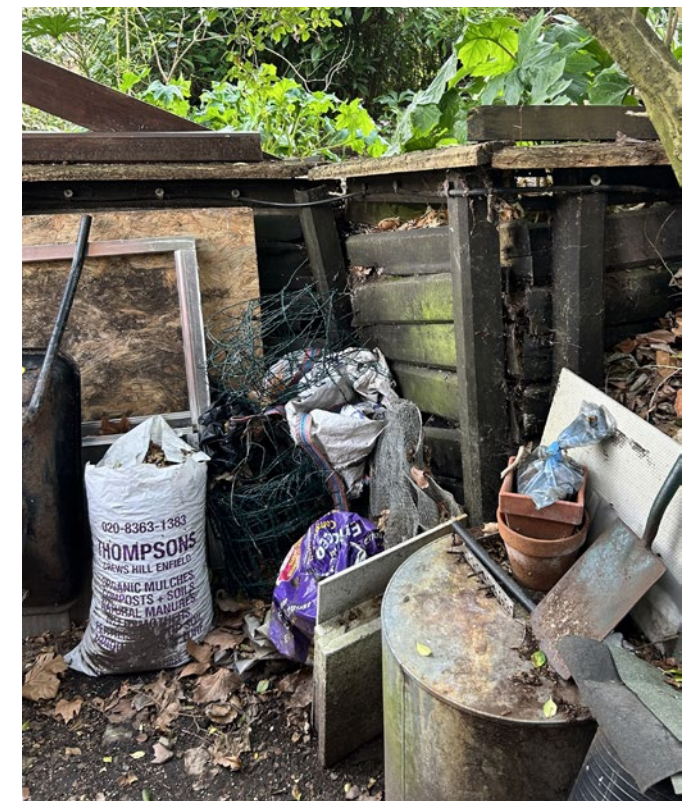
Image 07 | View dilapidated timber retaining wall to be replaced.
