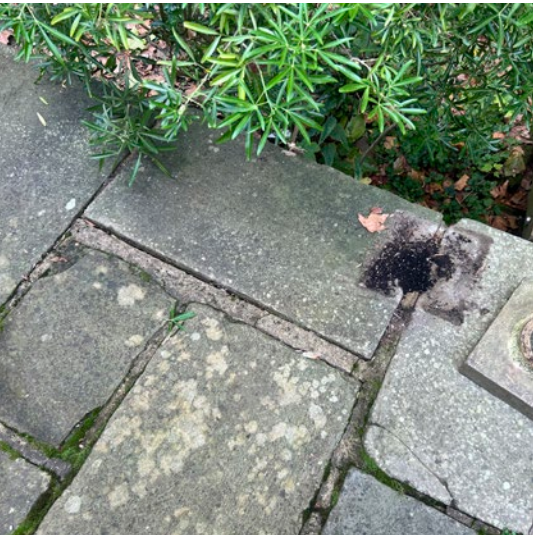
Terrace Stone | Existing stone slabs retained and supplemented with new reclaimed stone to match.
