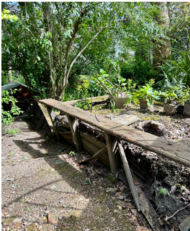
Image 04 | View of existing low-level timber retaining wall in poor condition.
