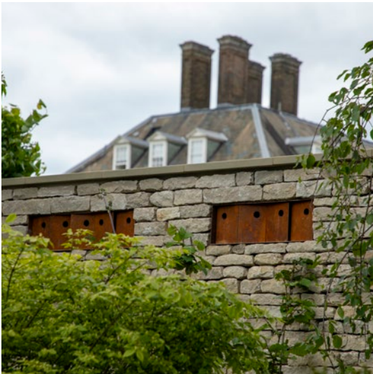
Retaining Wall Example | Example photo of wall constructed using Durlston stone with Luciano honed coping.
