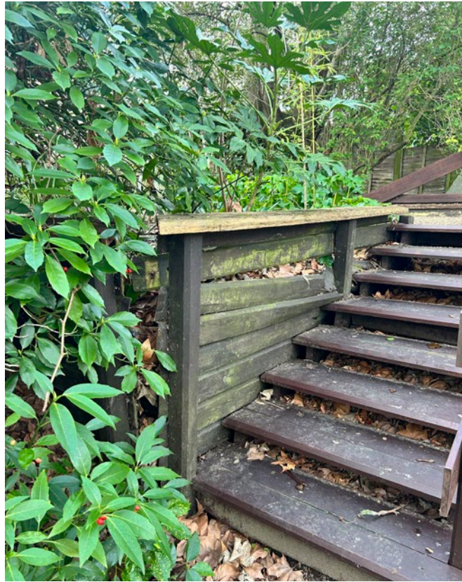
Image 09 | View of existing timber steps and failing timber retaining wall.
