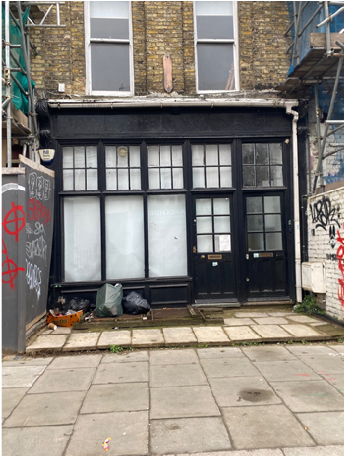
Historic shopfront with grille to basement lightwell in front
