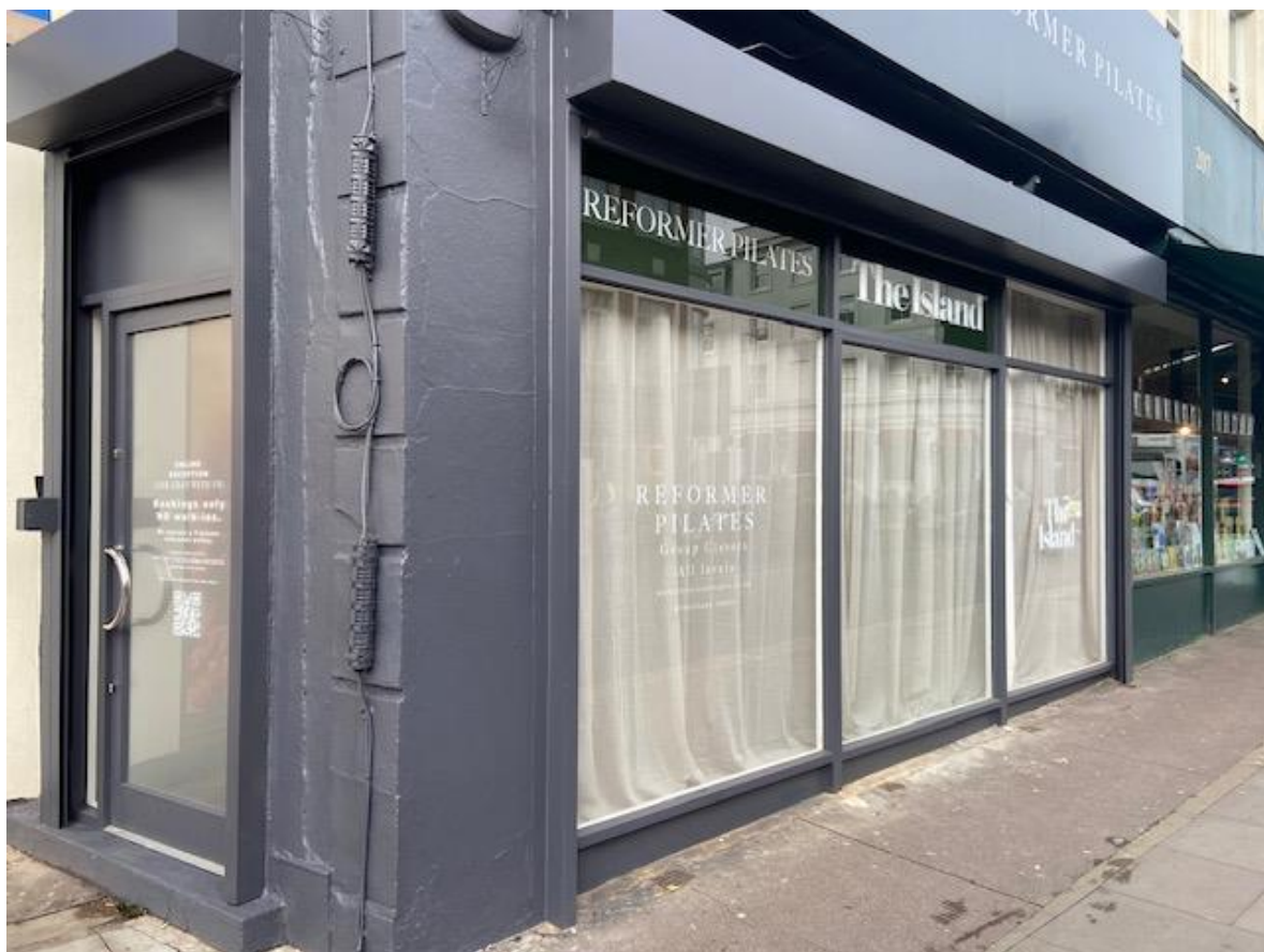
Figure 1 – Photographs of shopfront as built without planning permission
