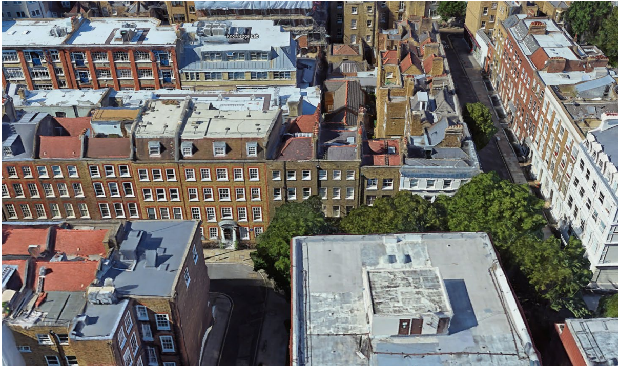
Fig.04: Existing building: 22 Great James St, showing streetscape around the corner of Northington St.
