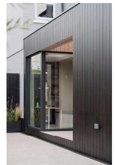
Examples of Powder coated aluminium cladding extension with Powder coated aluminium door
