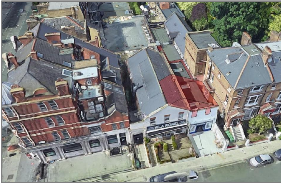
Figure 6. Aerial view showing proposed extension highlighted in red
