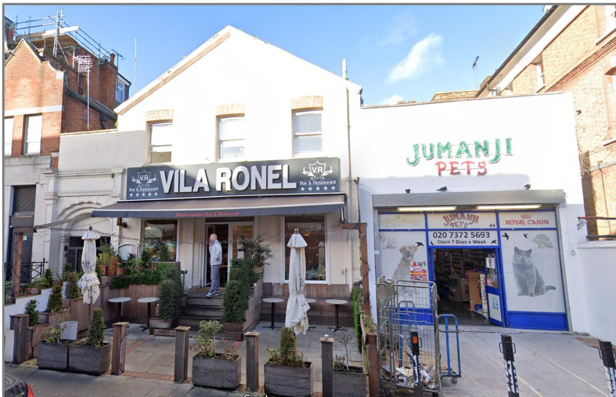
Figure 5. View of the site from street level
