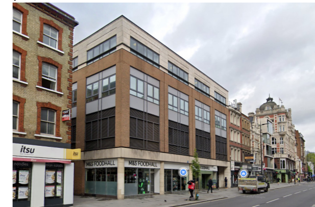
Louvre present on first floor in the existing building
