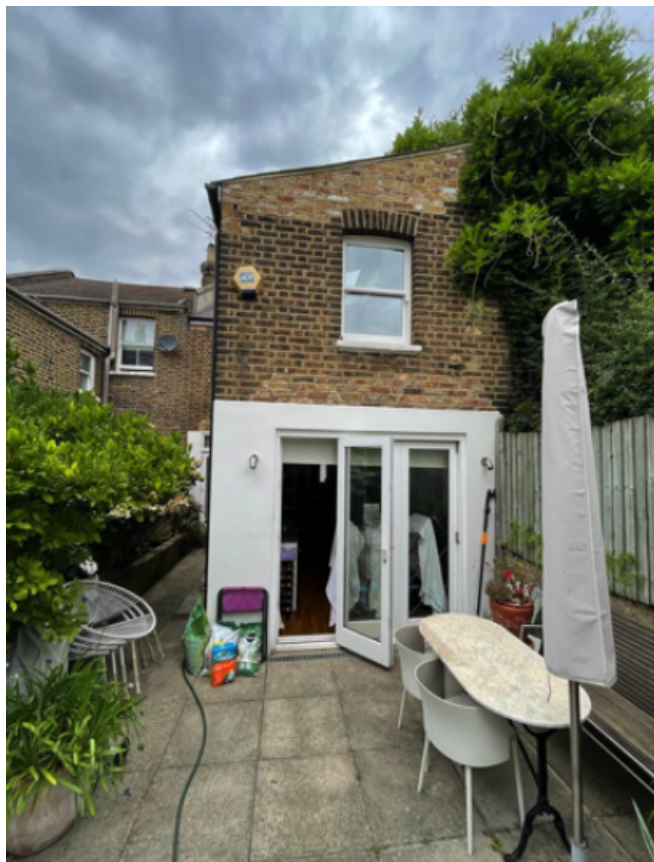
2. View of rear elevation
