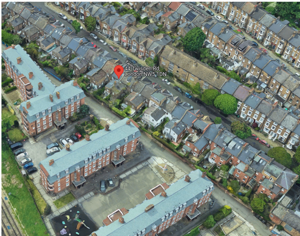
4. Bird's eye view of the site looking west
