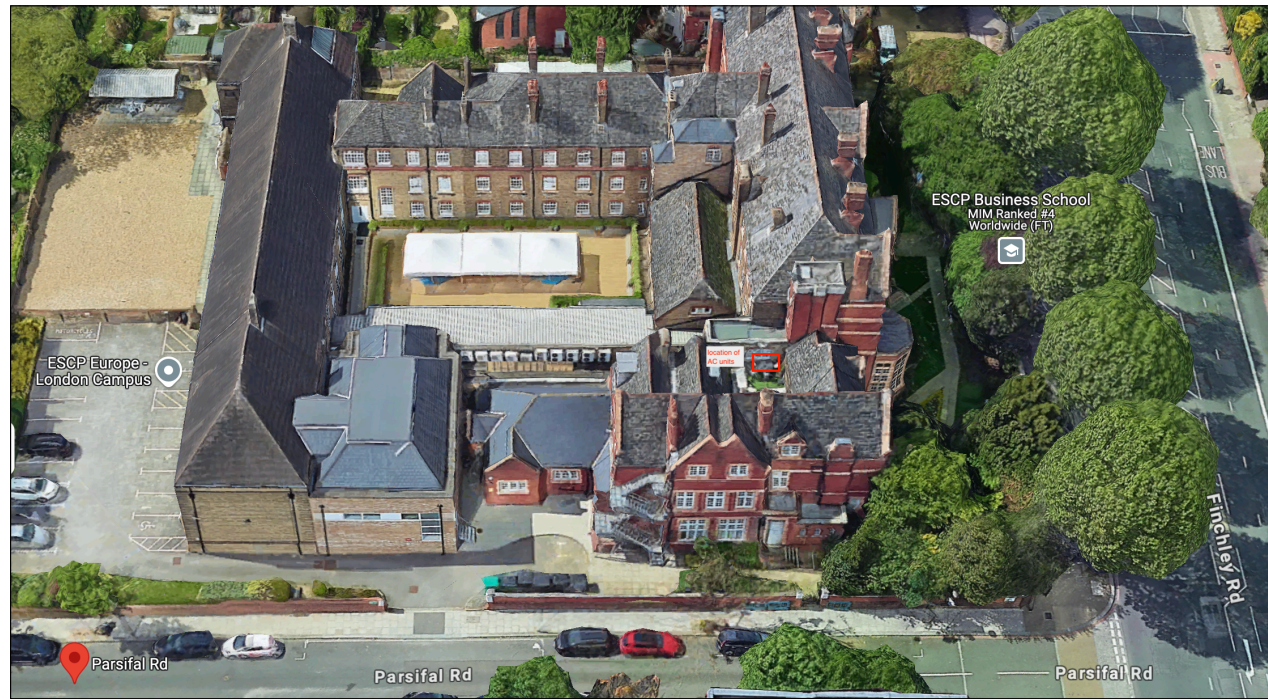
AERIAL VIEW FROM PARSIFAL ROAD
