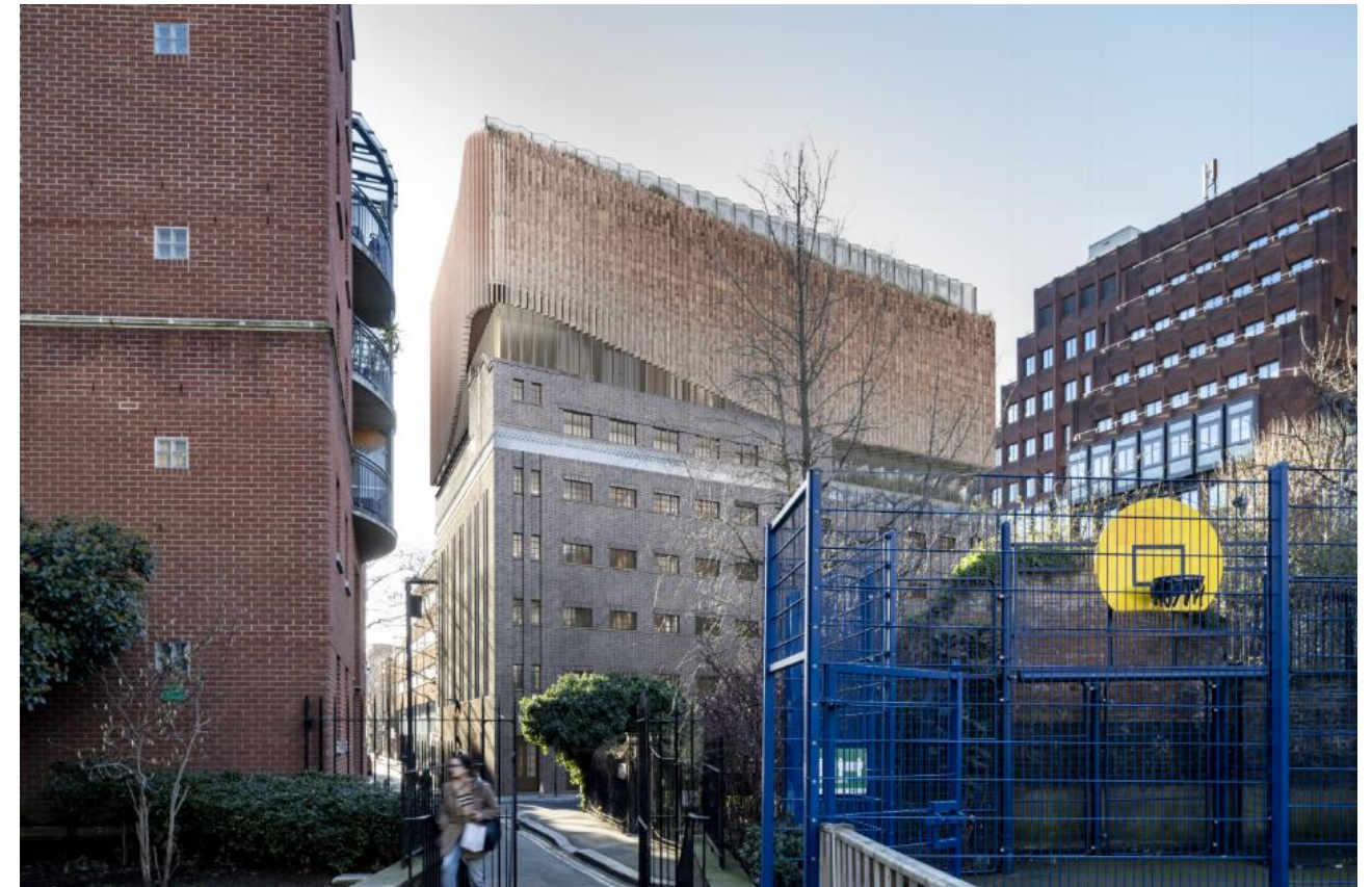
Figure 2: View from Shaftesbury Avenue of Proposed Development. (Source: SPPARC, Date received: 15 th December 2025).
