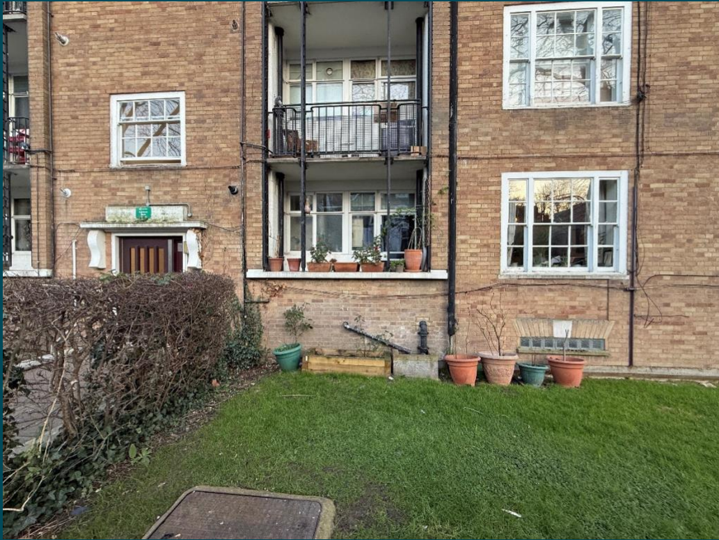
Appendix 2: External rear elevation of application flat
