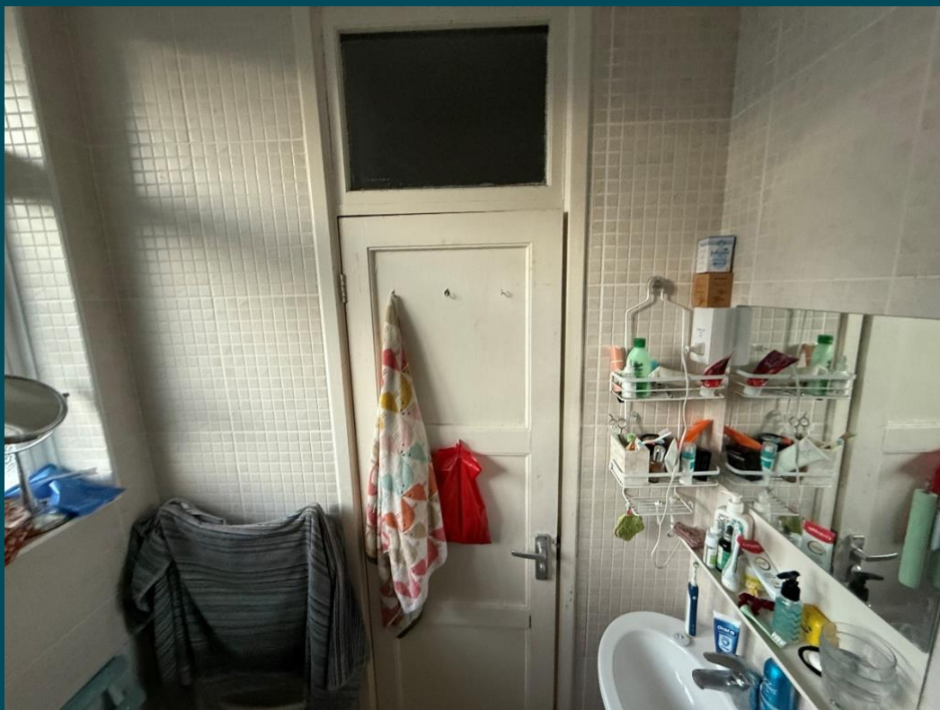
Appendix 5: Existing bathroom/ toilet wall (to be removed)
