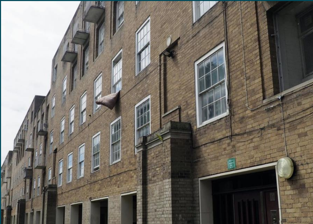
Appendix 1: Existing frontal elevation of Barn Field
