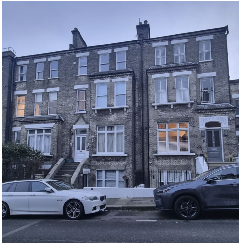
North West Facing front view with adjoining property N0.40 & N0. 44 from Denning Road
