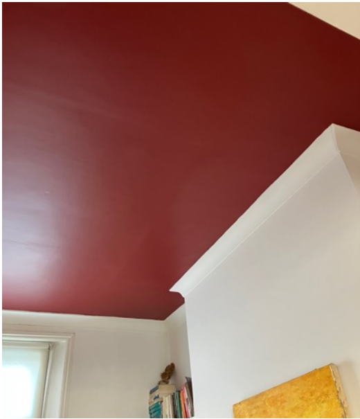
Ceiling and cornice rear room
