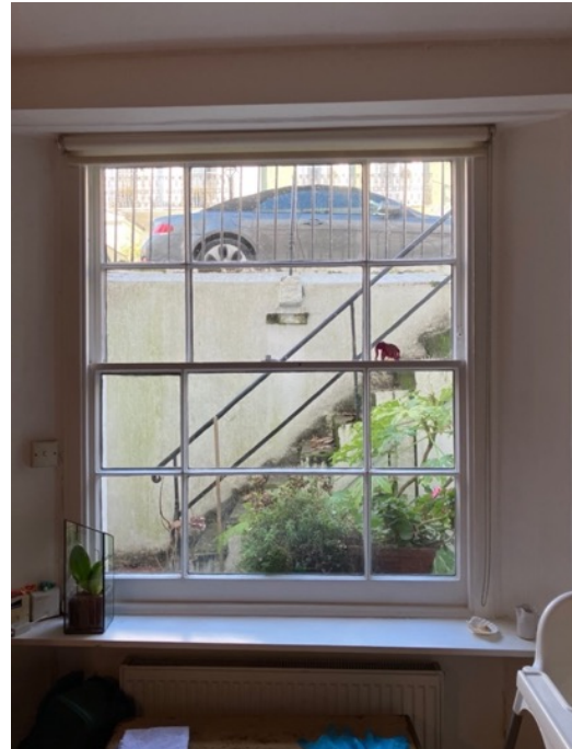
WB1 original sash (with modern cill)
