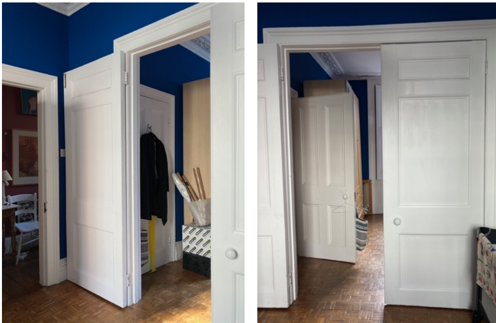
Double doors (DG4) fold back flat and DG3 seen beyond into rear reception
