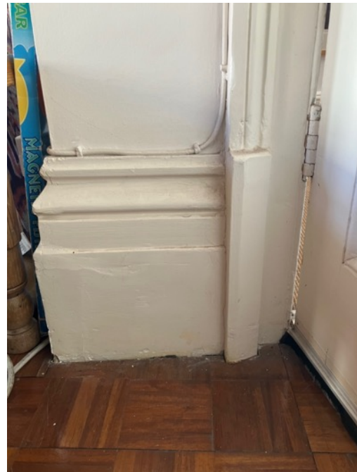
Joinery detail and flooring
