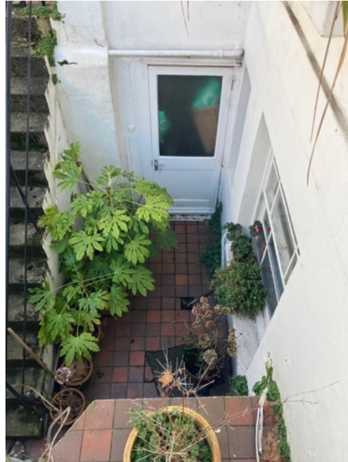
Quarry tile finish and storage spaces
