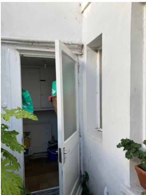
Modern openings to area DB1 and WB3
