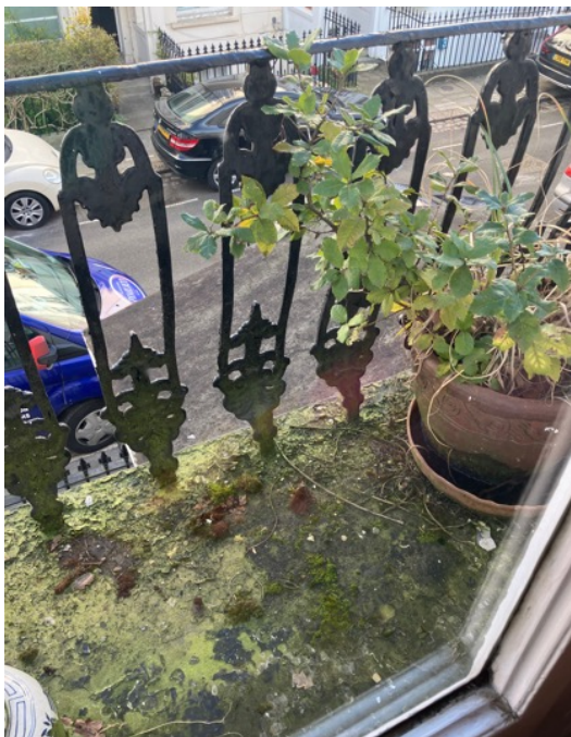
Balcony and casement condition
