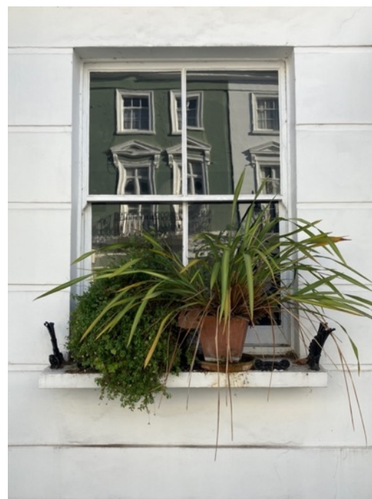
Ground Floor Window WG1
