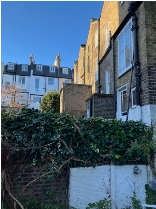
Boundary wall and trellis to no. 8
