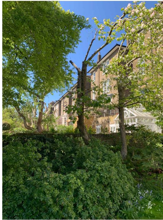
Garden wall with 135 King Henry's Road North Elevation
