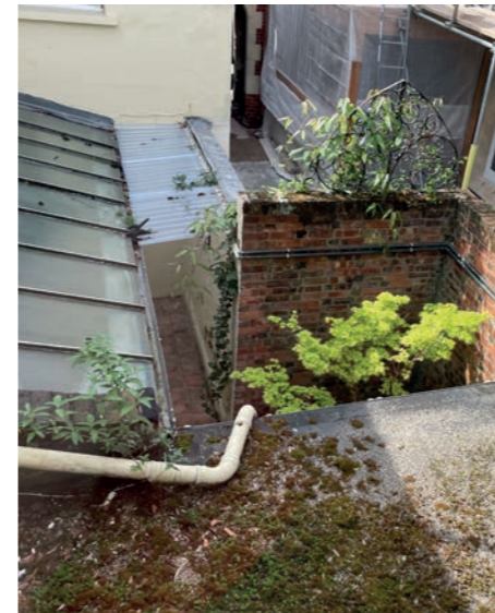
View from bedroom to front external courtyard
