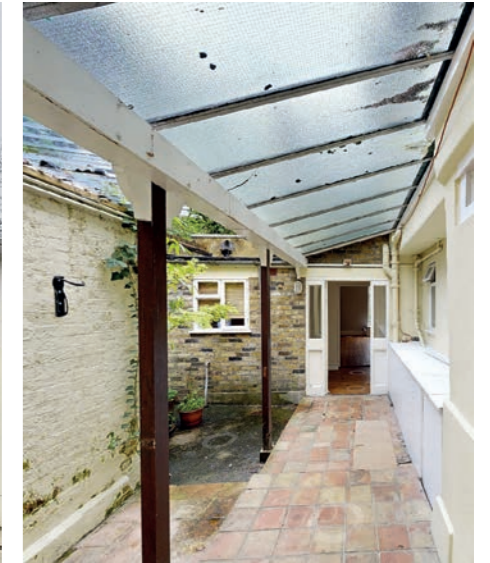
View through entrance passage to property
