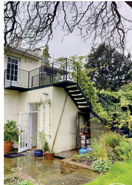
Current condition of extension.
