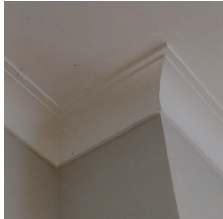
Existing Condition: Plain, modern coving
