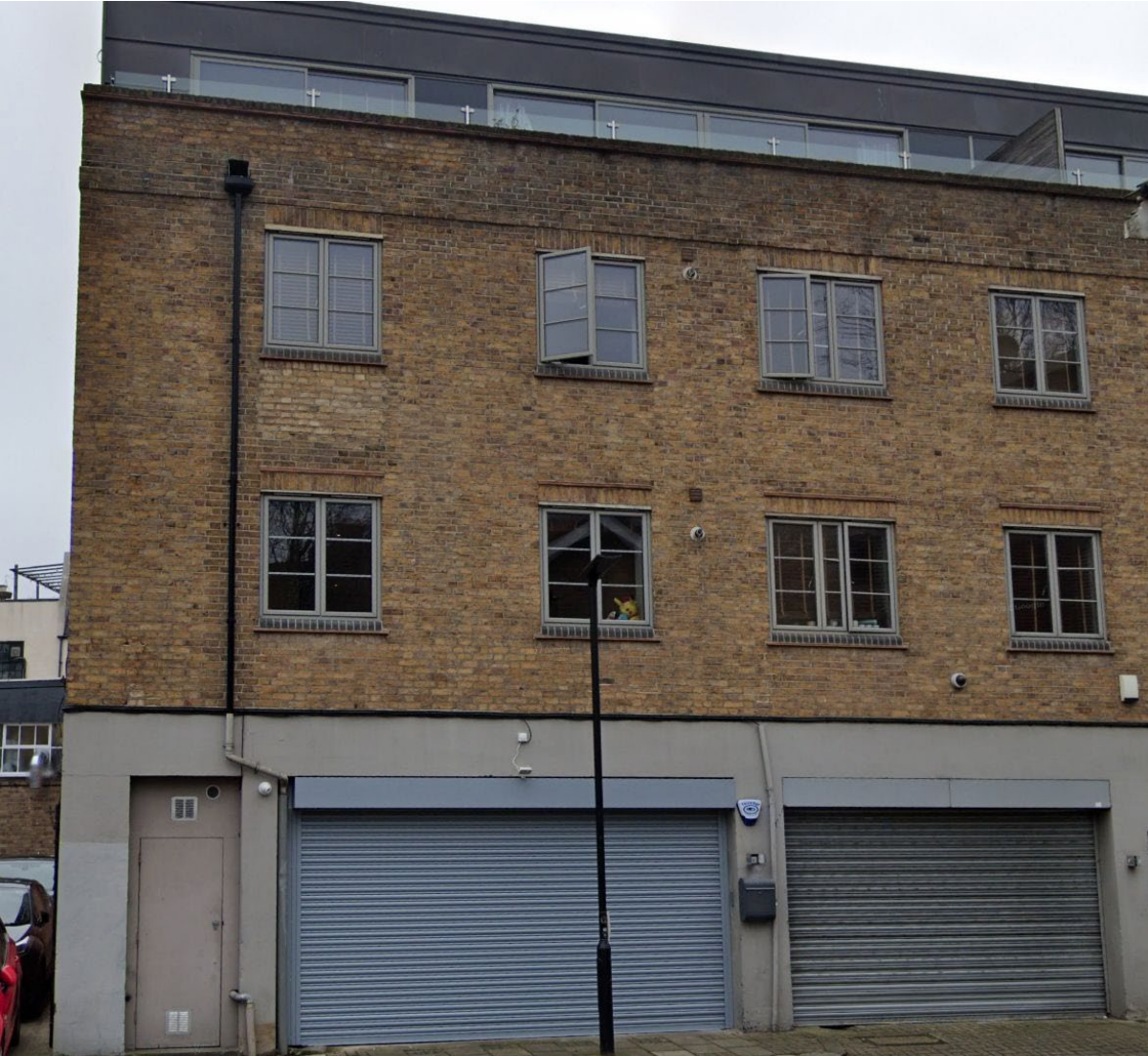
Neighbour Building_2 Ferdinand Place Materials- London Stock Yellow Brick, Light Grey Window / Door Frames
