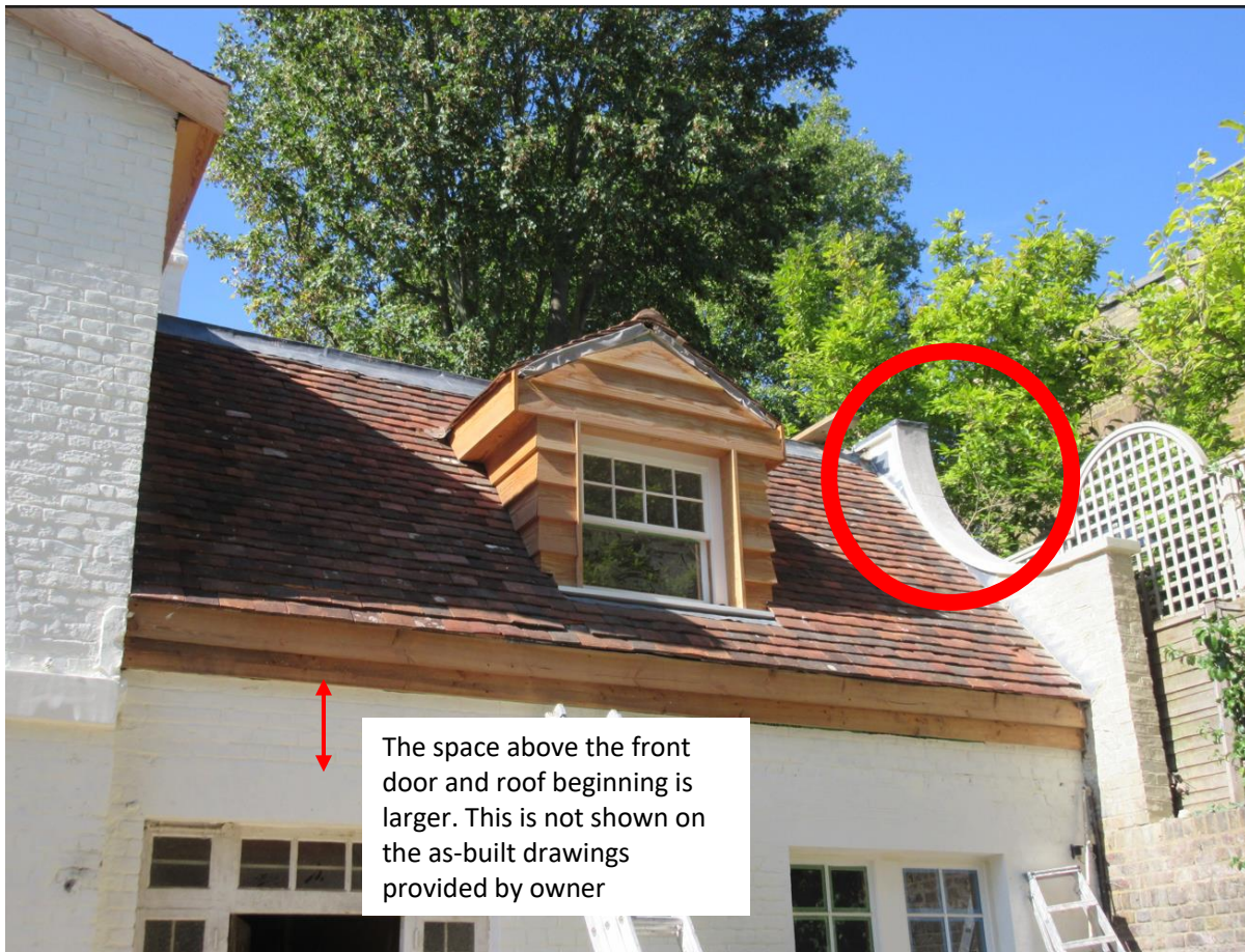
Figure 21. Site photograph showing the as-built roof on 14 th September 2023. This shows the ground floor height has been increased as the position of the eaves of the new roof has altered. The red circle shows the as built position, pitch and height of new roof.
