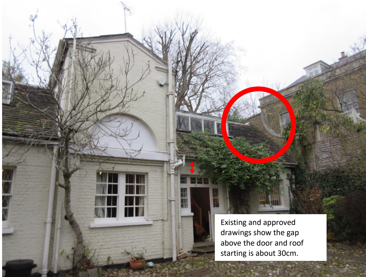
Figure 20. Site photograph showing the pre-existing front elevation and the gap between the top of the front door and eaves of the roof. The red circle shows the relationship between the roof and the end wall.
