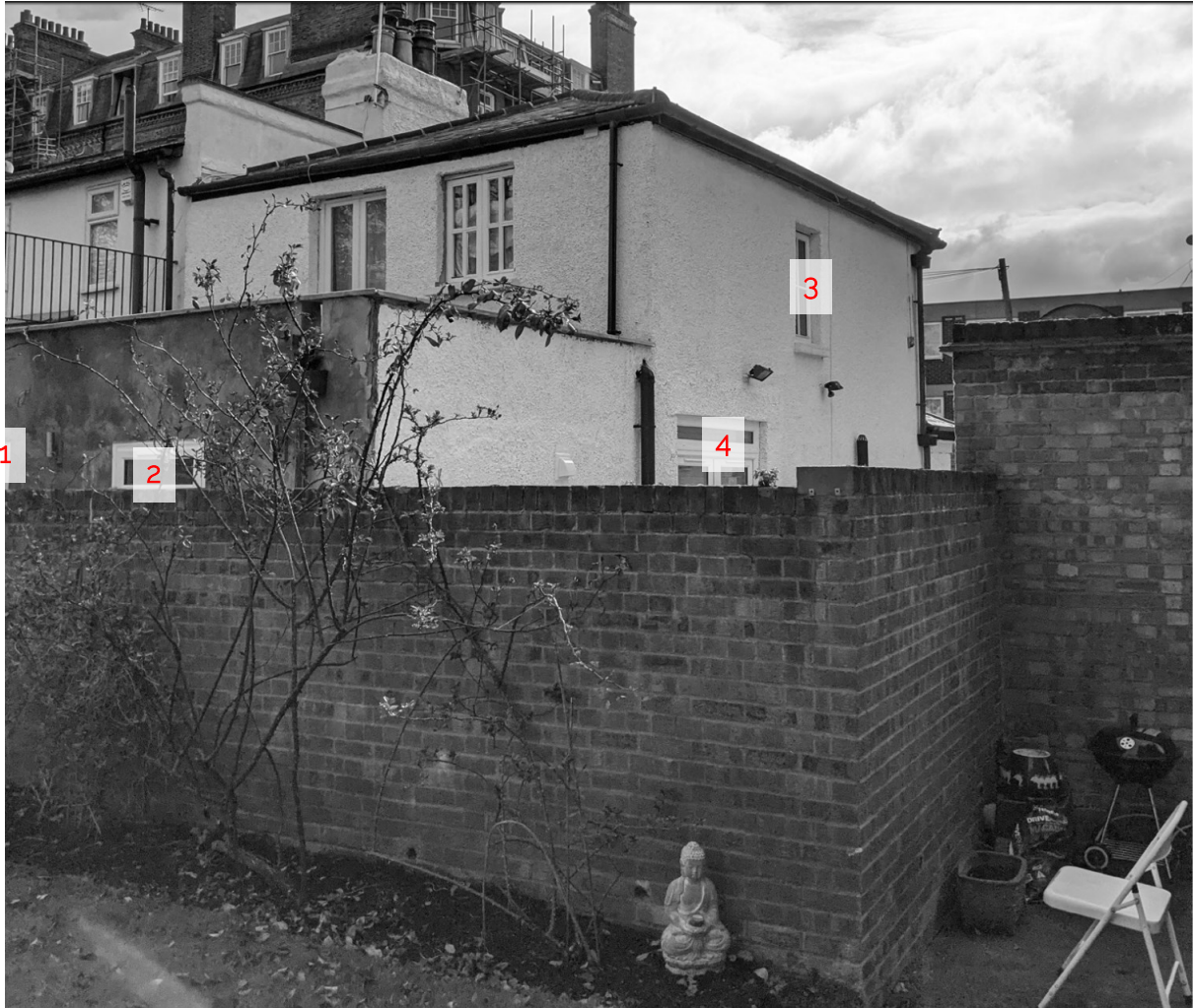
13 West Cottages, Rear Elevation
