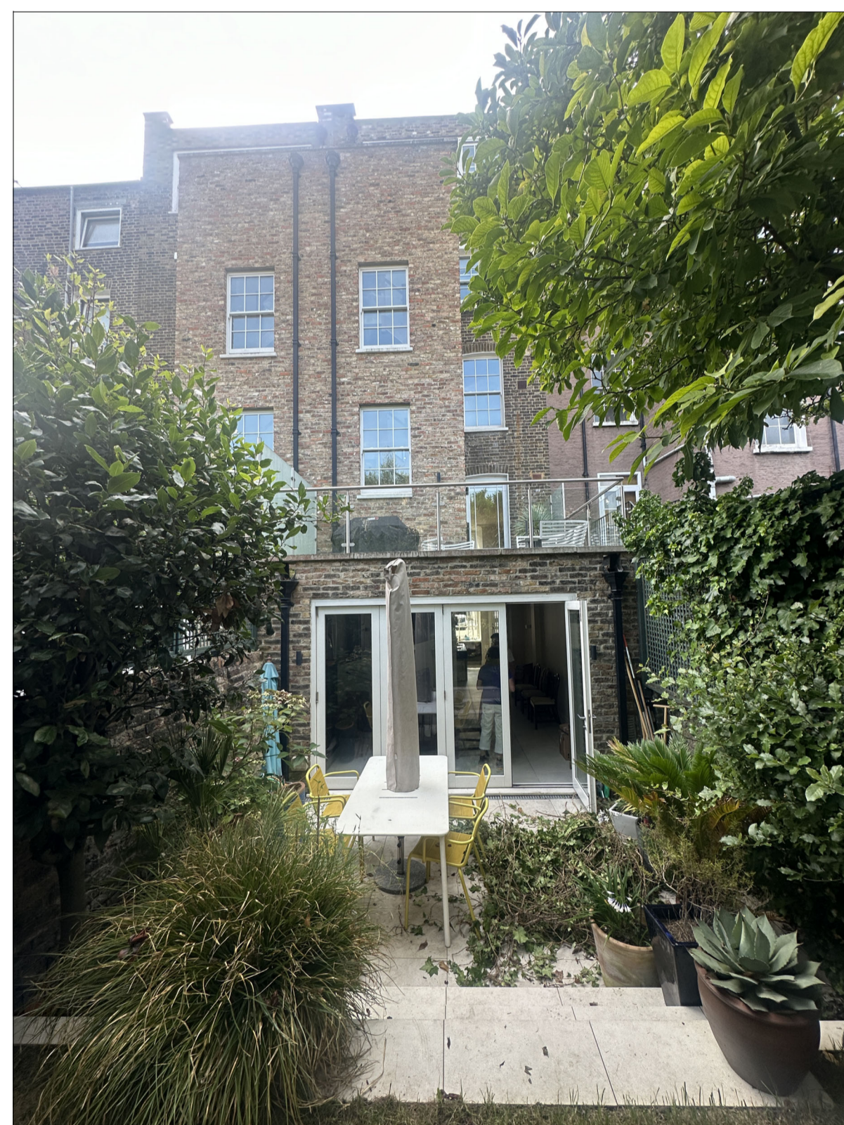
03 VIEW OF THE TERRACE
