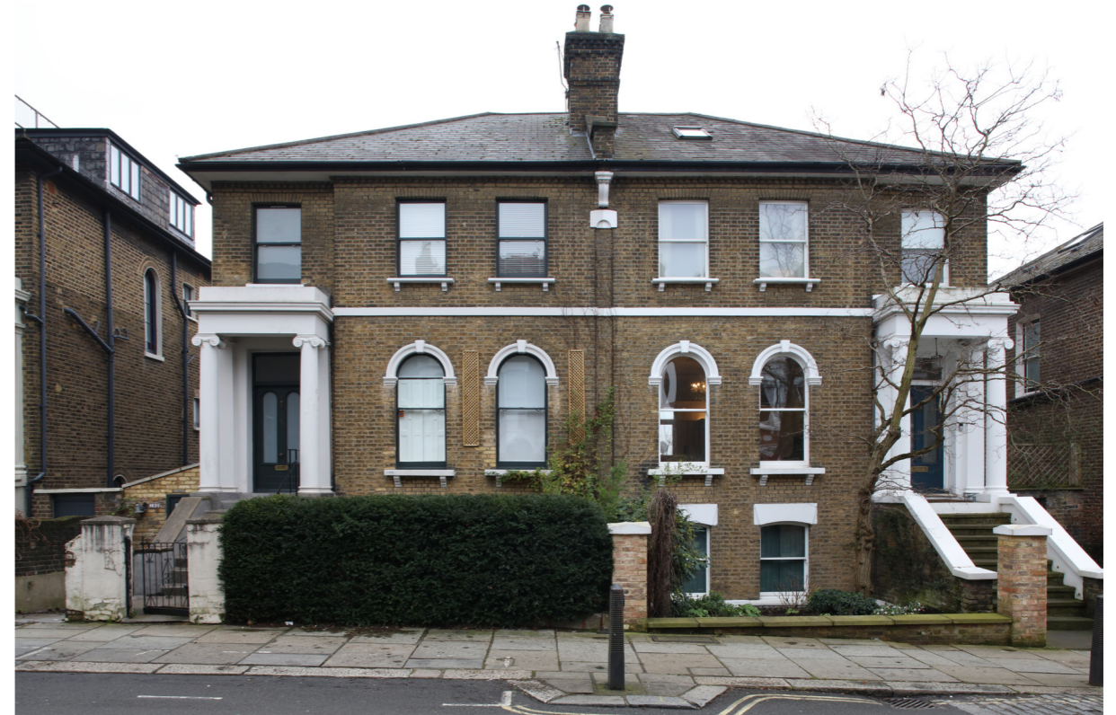
100-102 Chetwynd Road Street Facade
