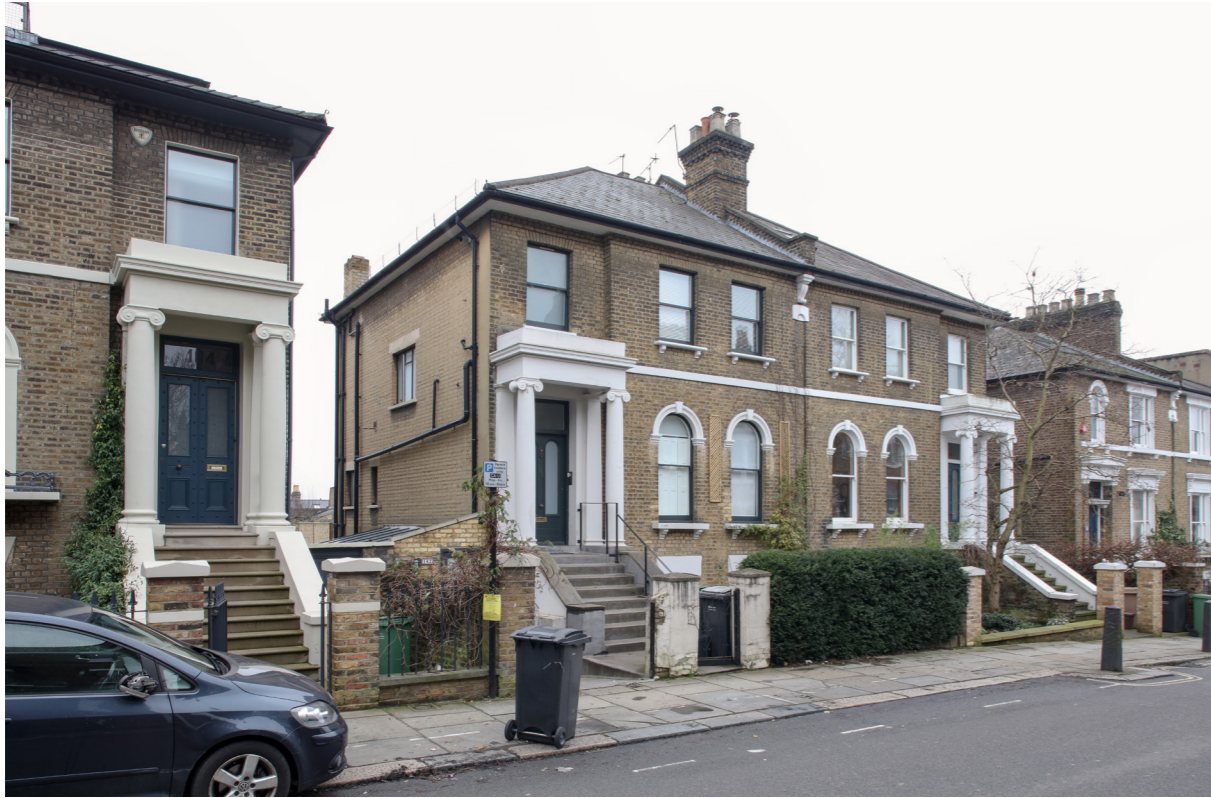
102 Chetwynd Road (the Site) Oblique View
