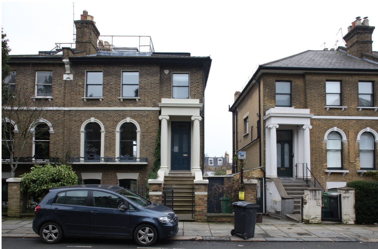
102-104 Chetwynd Road Street Facade
