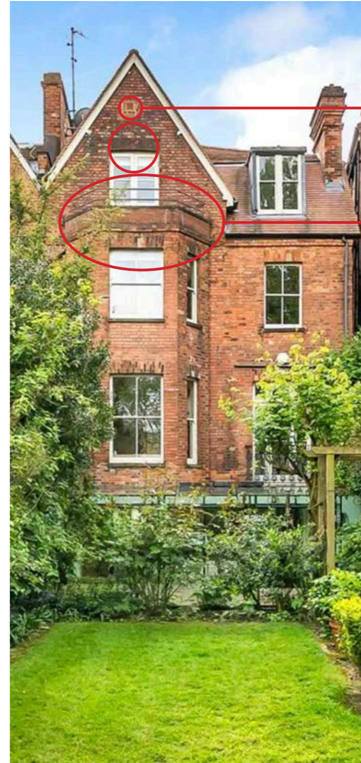
This lintel has dropped slightly, area requires repair and repointing.
