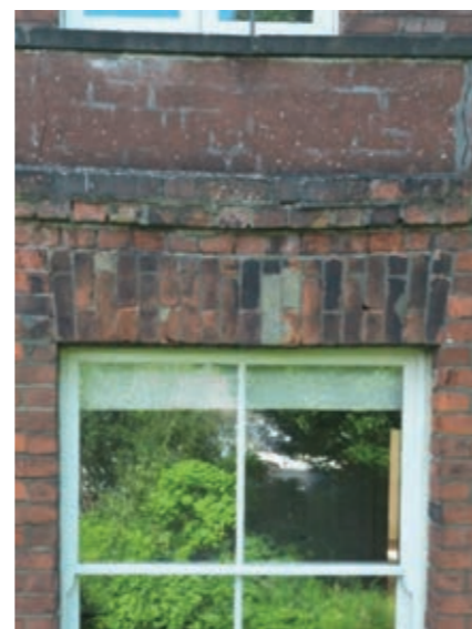
This lintel has dropped slightly, area requires repair and repointing.
