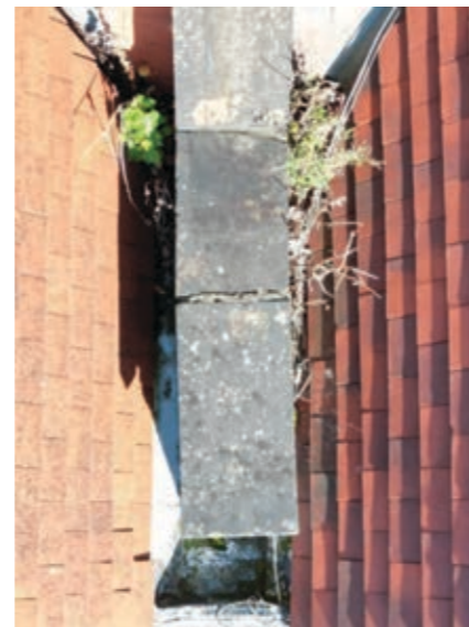
Detail of blocked gutter to the rear of the property, this requires clearance.
