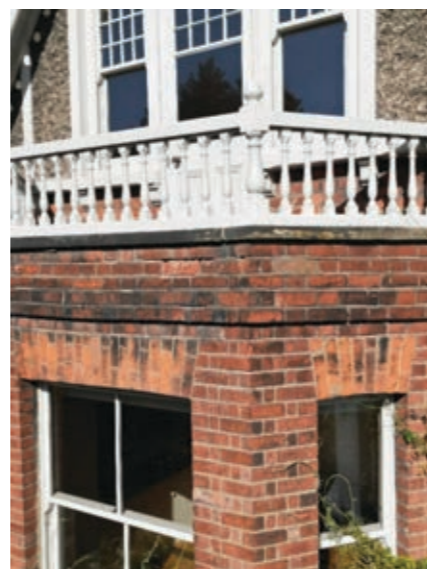
Detailing of open mortar joints.
