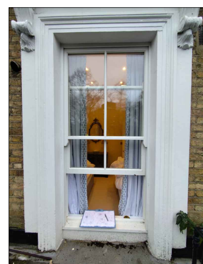
Existing window with matching Timber Sash and double glazing.
