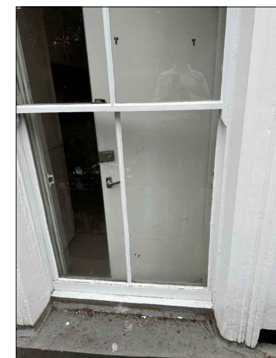
Pre-Existing window with Timber Sash and single glazing.
