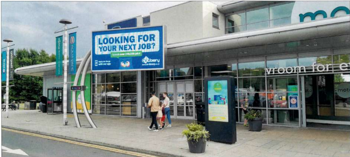
Picture 10.3 – Digital displays ground mounted, and on purpose design structure.
