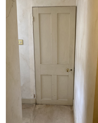
D L.01 Existing door to bathroom
