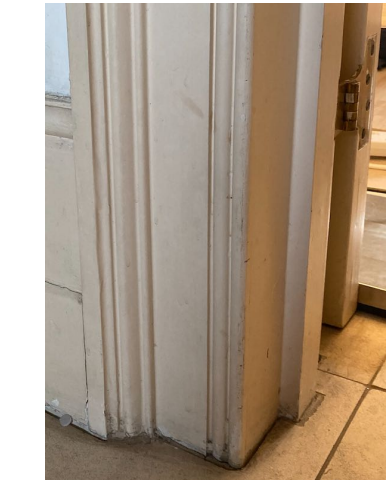
Architrave to match the existing w 125mm
