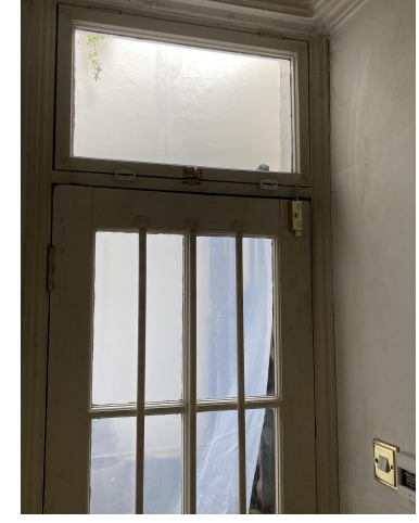
LGF Architraves b=65mm to match the existing
