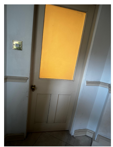
D G.01 Existing bathroom door
