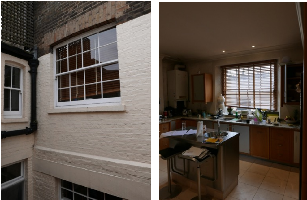
Plate 16 (left). Kitchen window from top of courtyard steps. Plate 17 (right). View towards window from inside kitchen.
