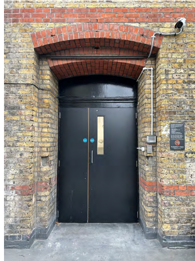
Existing Access Point
