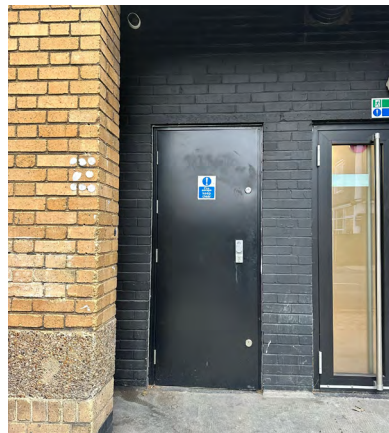
Existing Access Point
