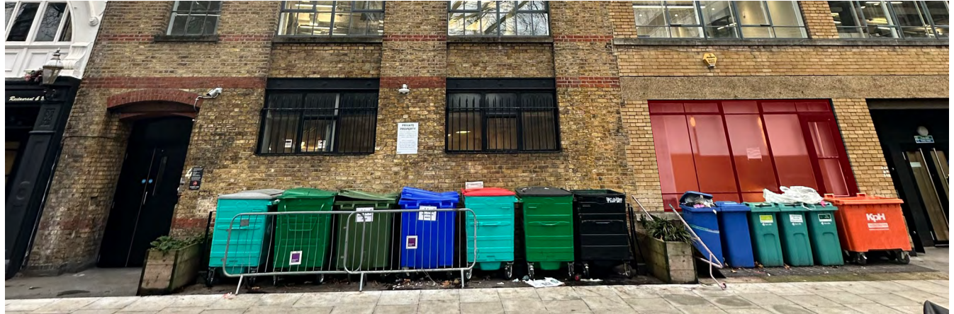
West Elevation Replaced Glazing
