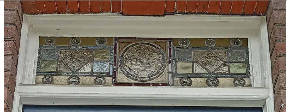
Fanlight detail of existing front door. Refurbished fanlight panel (with float glass) to sit on external facing side of the treble glazed unit, with outward facing leadwork.
