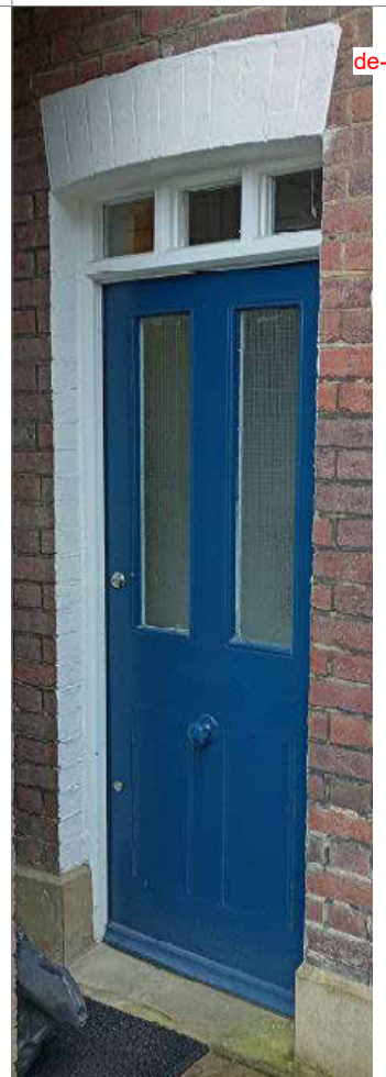
Lower ground floor door
