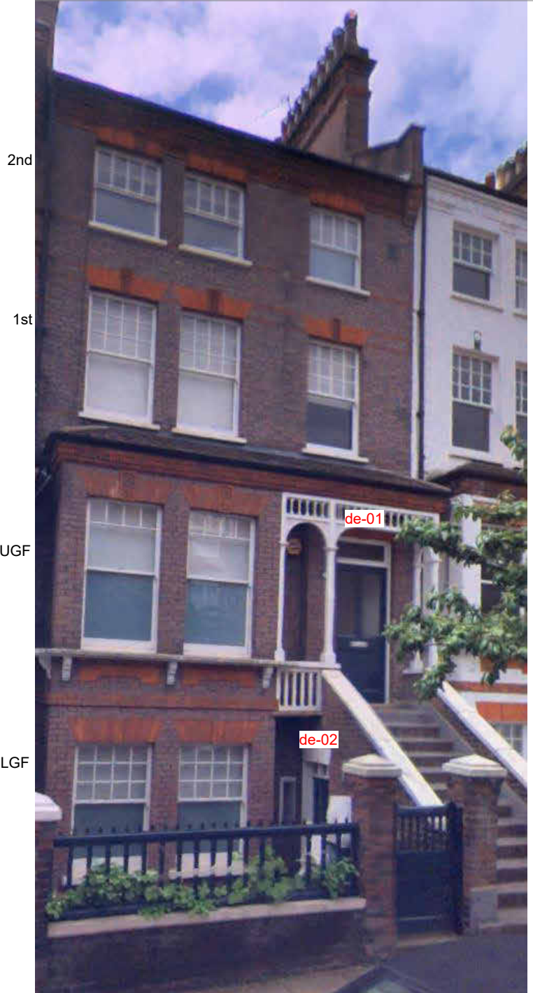
Main front elevation overview
