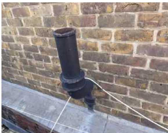
RPT-Figure-22: Soil pipe to the south had been encapsulated in masonry
