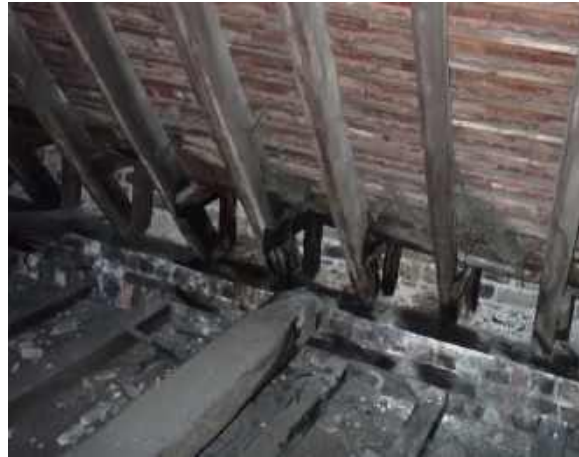
RPT-Figure-7: View of eastern parapet wall
