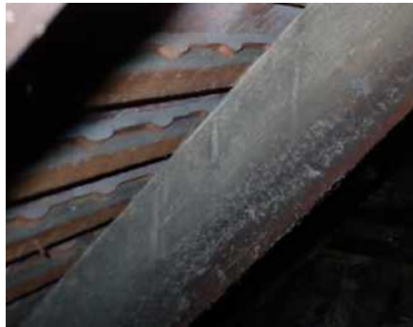
RPT-Figure-25: Bracker's marks were worn in some areas though still visible
