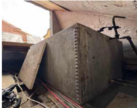
RPT-Figure-17: Cistern installed within roof access point, likely Victorian in nature
