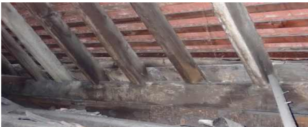
RPT-Figure-12: View of structural arrangement at southern, hipped pitches
