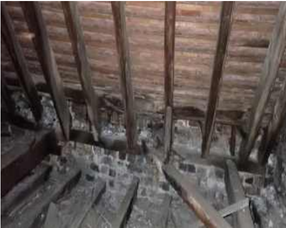
RPT-Figure-6: View of western parapet wall
