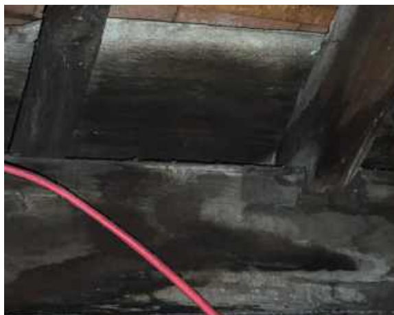
RPT-Figure-27: Differing jointing methods noted in localised instances
