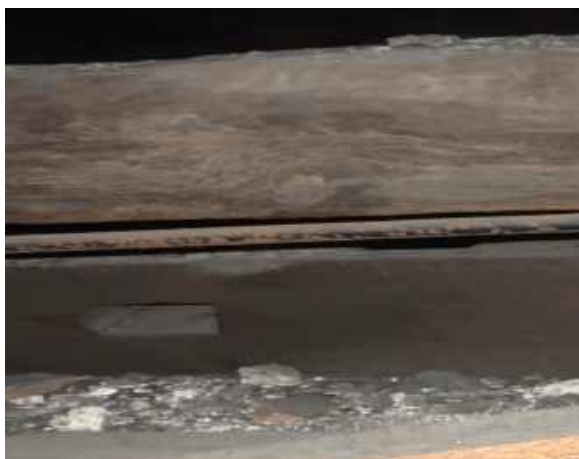
RPT-Figure-28: Different generations of timber were noted within roof voids
