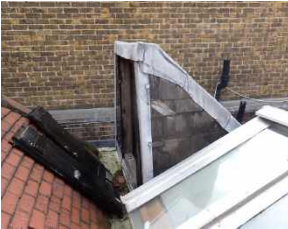
RPT-Figure-16: Slate used to dress cheeks of roof access point
