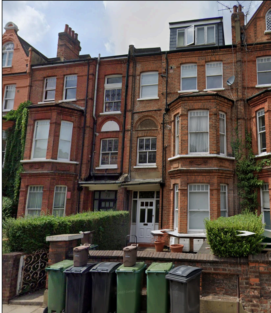
3.1 Above a view of the current site from the road
